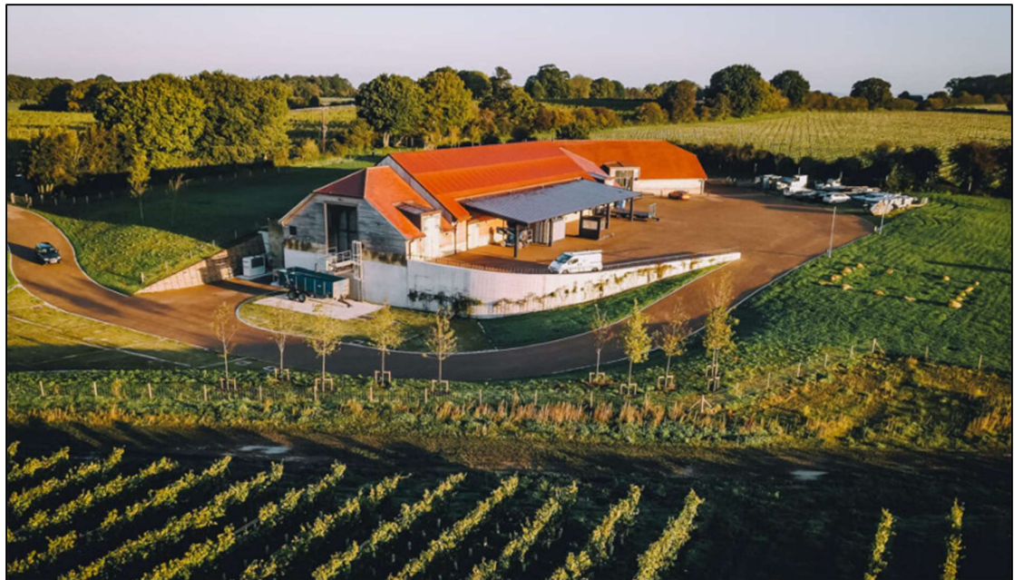
Figure 5 - Image of existing pressing centre
