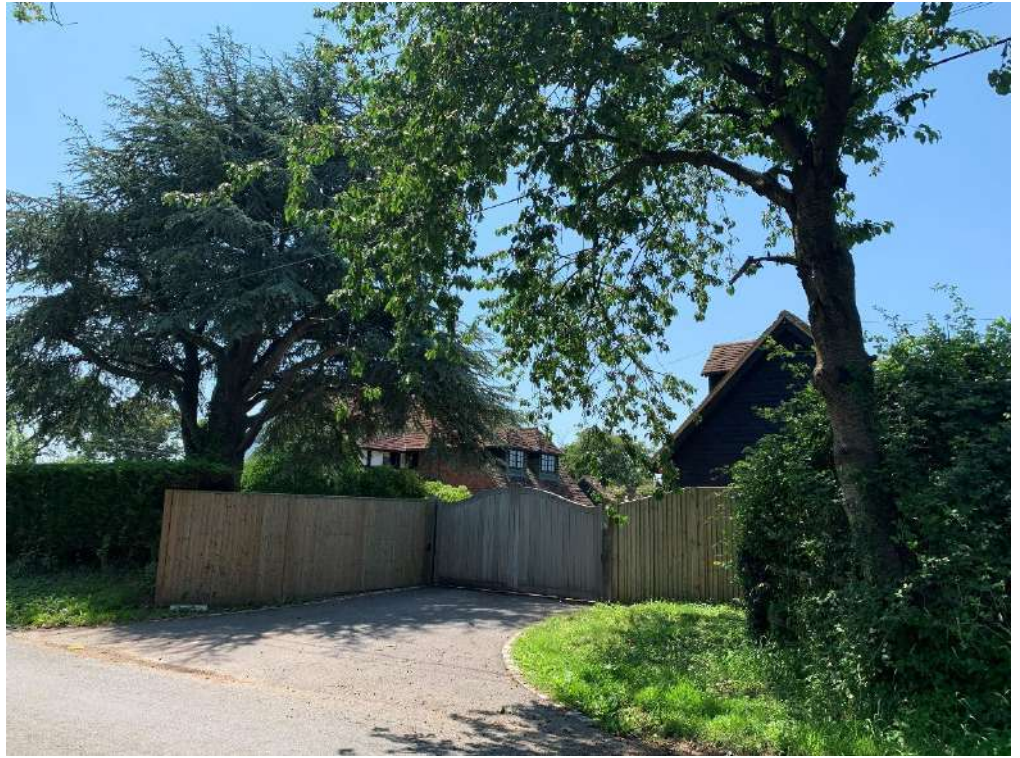
Plate 5 West view of Huntleys (NHLE 1354117, Grade II) from along Broadford Bridge Road
