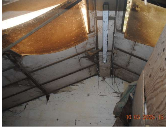
Photograph 8: A view of the roof within the stable unit in the rear of the building (northern extent).
