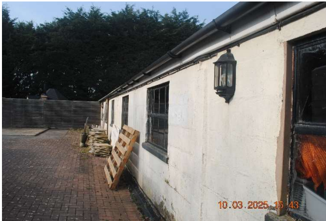
Photograph 3: The western elevation of the building.
