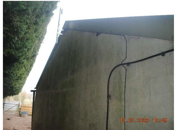
Photograph 4: A view of the northern gable end.
