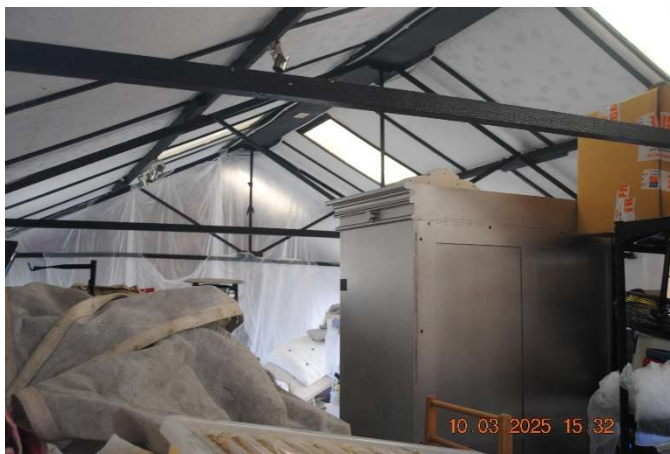
Photograph 5: A view within the central section of the building used for storage.
