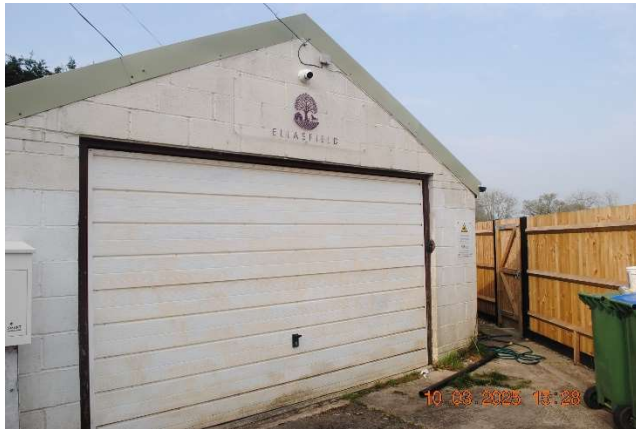
Photograph 1: A view of the front (southern) elevation of the building. The building was well sealed.
