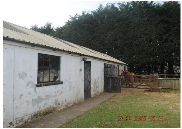
Photograph 2: A view of the eastern elevation.
