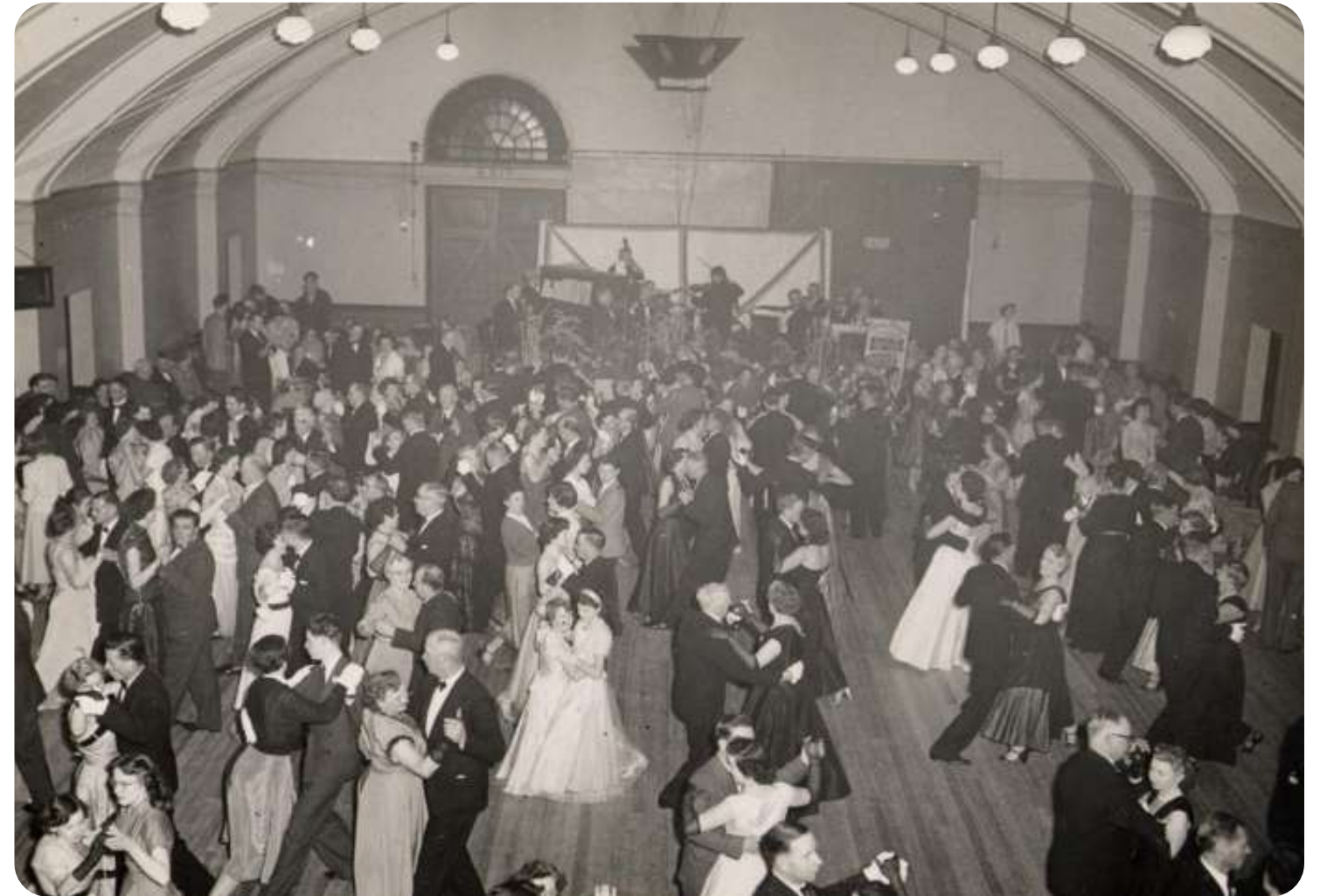
The main hall is the centre piece of the building. Through the introduction of new building services under this application, the hall will be provided with modern and compliant standards of ventilation allowing for continued effective use.
