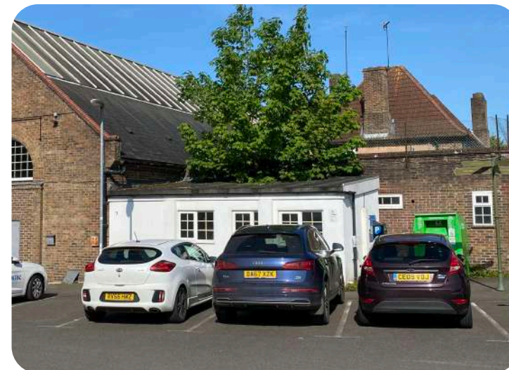
Existing toilet block to rear of the building proposed to be re-built as Green Room to serve the hall.
