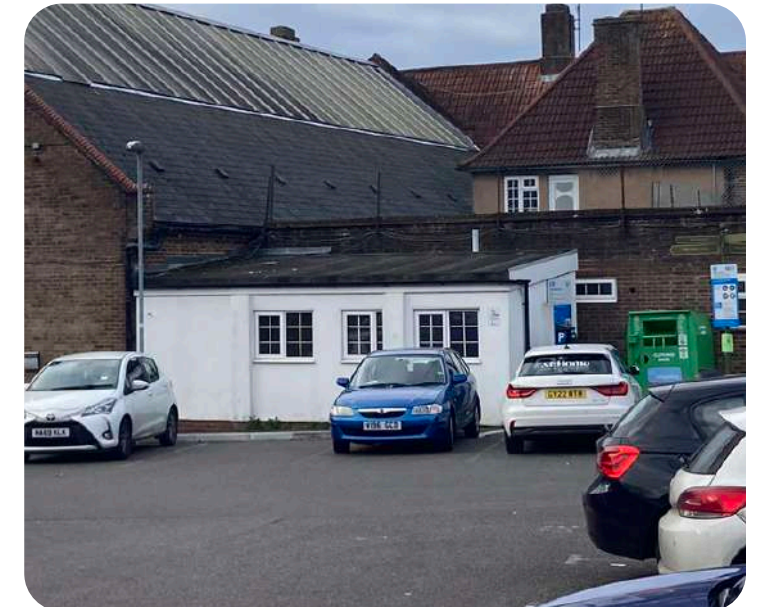
The non-original and poor quality toilet block will be rebuilt in materials to match the existing building.
