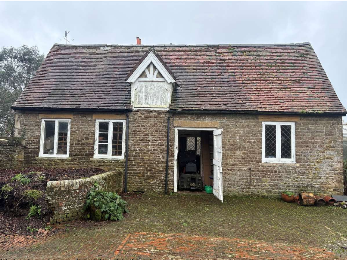
Main elevation to the old stable block
