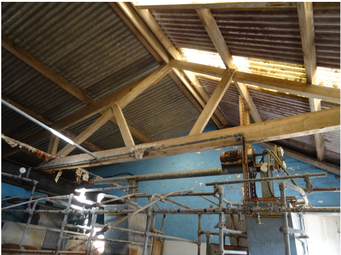
Internal Building No.2
