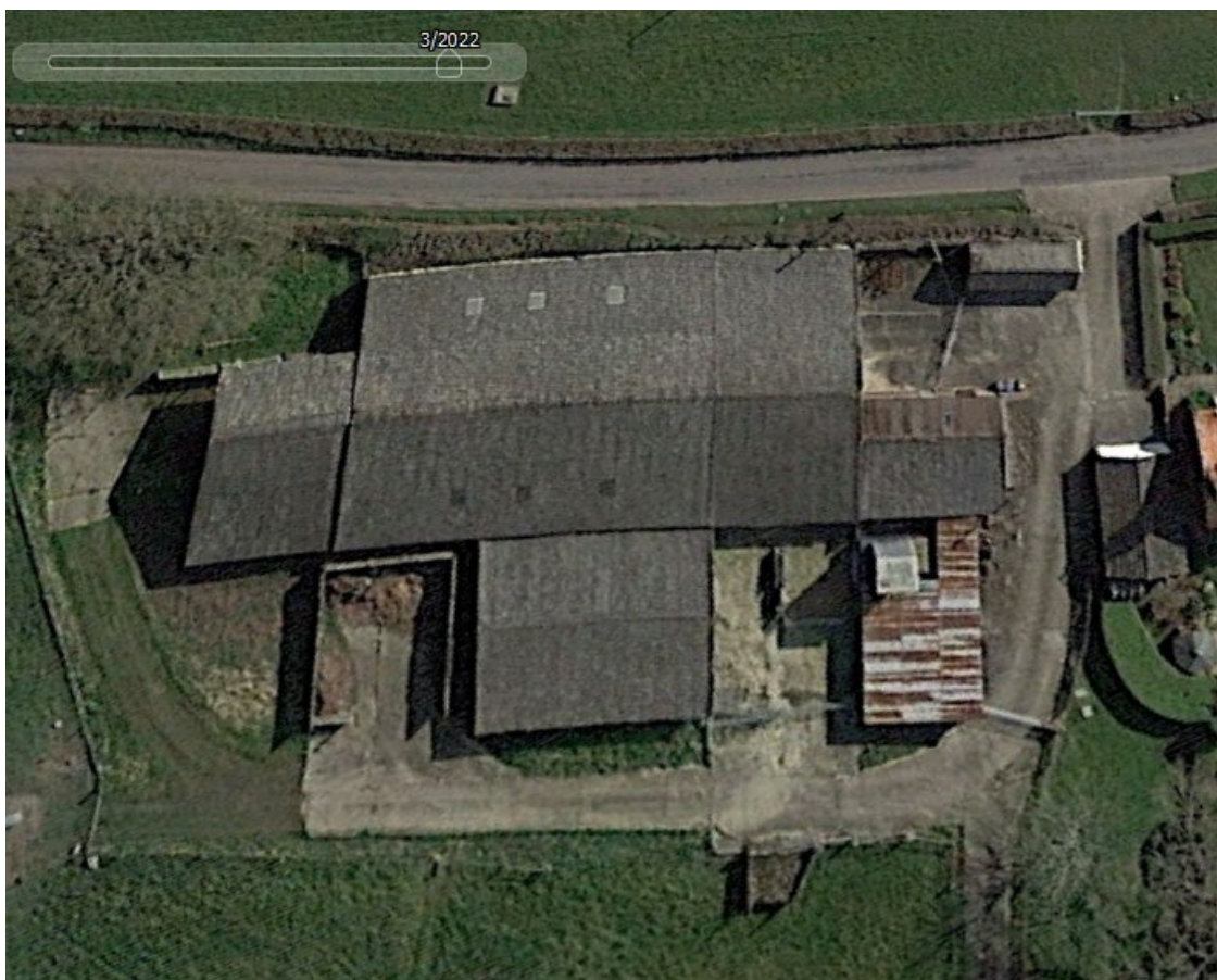
Figure 4.1 – Google Earth Image of the rear of the application buildings (March 2022)
