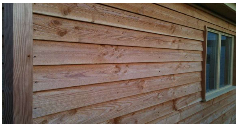
HORIZONTAL TIMBER WEATHERBOARDING
