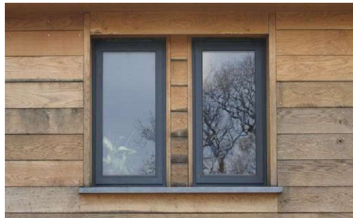
ALUMINIUM FRAMED CASEMENT WINDOWS
