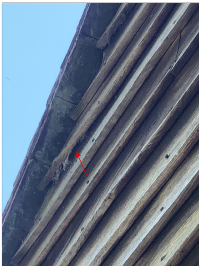
Photograph 4a (left) and 4b (right). The gap under timber cladding on the western elevation (left) and the interior of the void (right).
