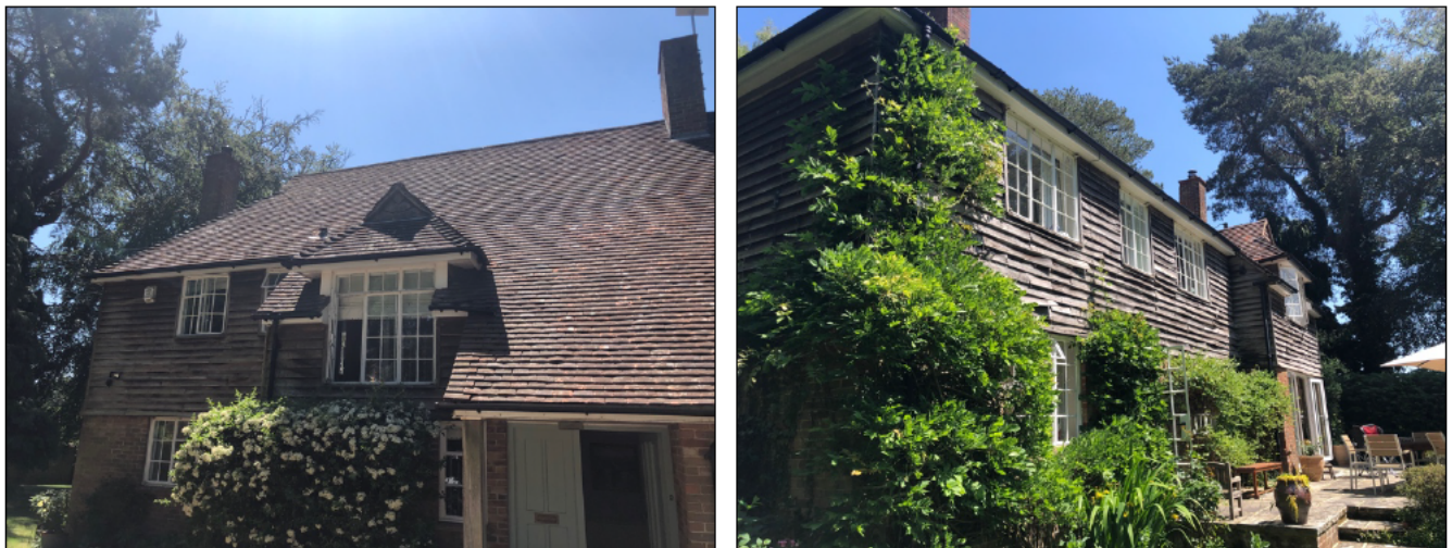
Photograph 1a (left) and 1b (right). The northern elevation (left) and the southern elevation (right) of the property.
