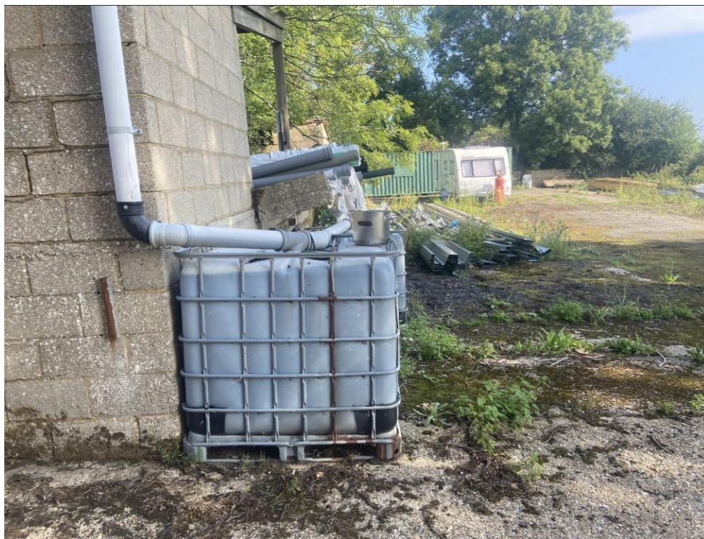
Photo 8: Downpipes and IBC were noted
