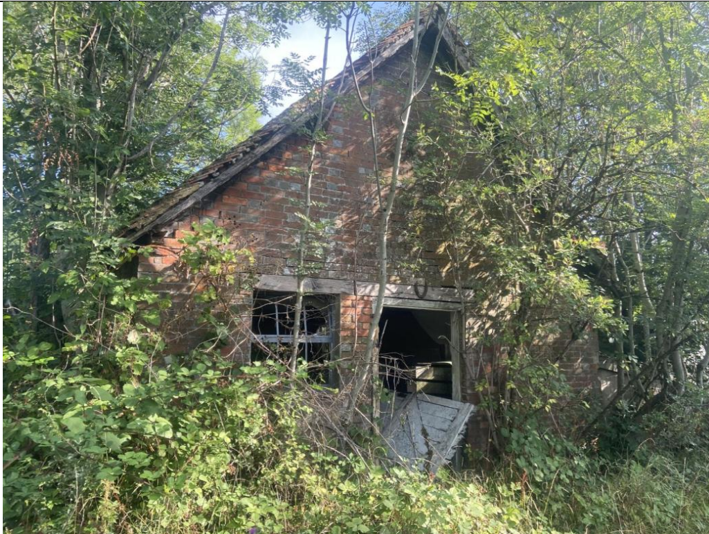
Photo 2: Pitched roof building and brick walls were noted
