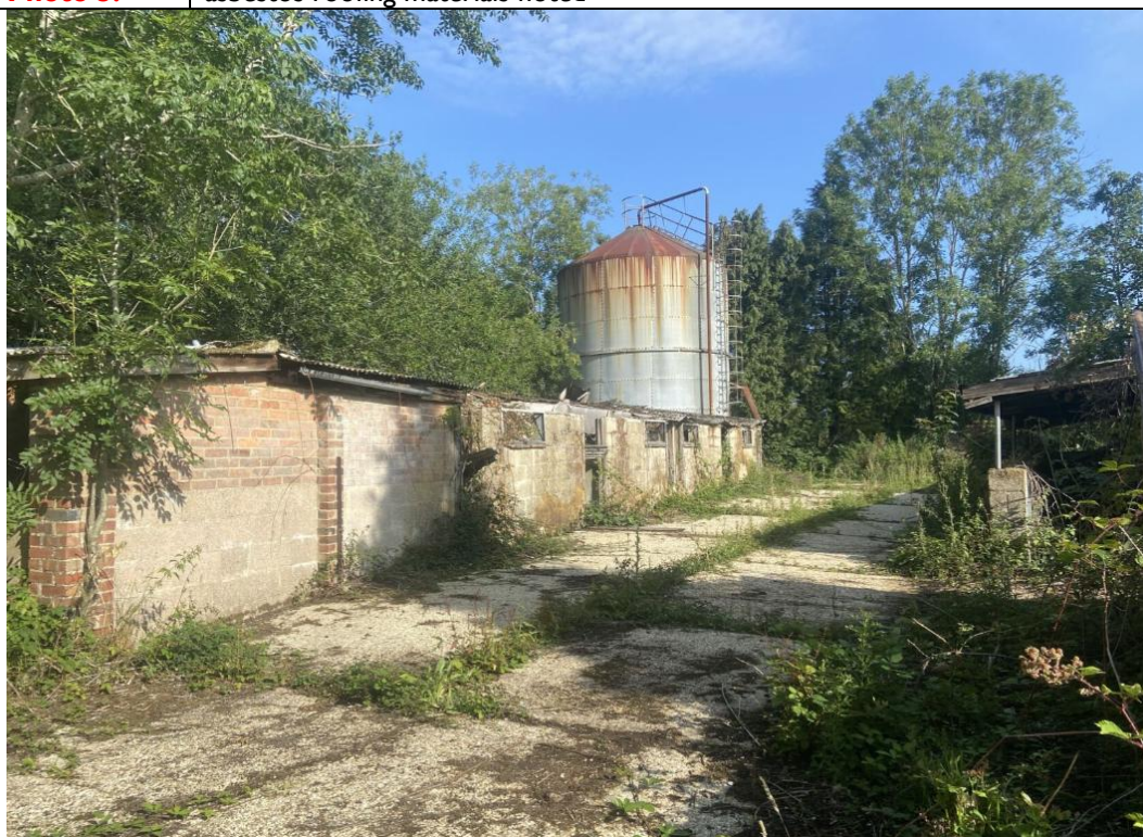
Photo 4: Metal silo was noted
