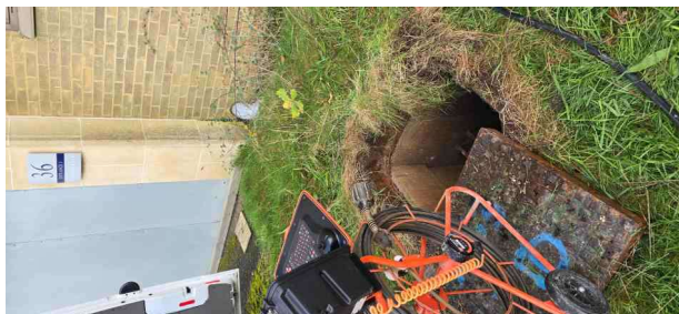
MH63X_84e43519-7d21-40aa-bcb9-b75b2af84fb4_20241125_142650.jpg, 00:00:01, 0.00 m Start node, manhole, reference: MH63
