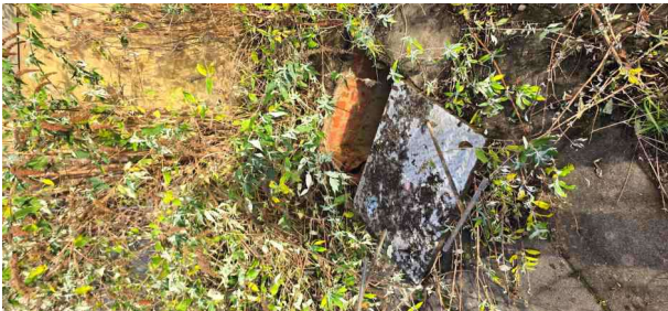
MH29X_70c4b88e-c05f-4202-9809-390d6086d4fd_20241125_113035.jpg, 00:00:47, 7.64 m Finish node, manhole, reference: MH27
