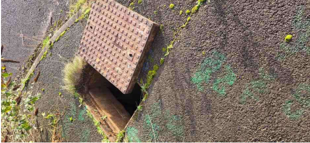
MH32X_84aef4aa-2e4e-4b57-8957-3d9b8e573ac4_20241125_105257.jpg, 00:00:01, 0.00 m Start node, manhole, reference: MH31
