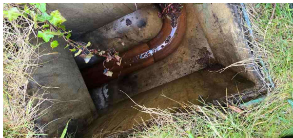
MH64X_d5373b3c-21a3-474c-b060-ec25bf1d1ca6_20241125_142625.jpg, 00:00:01, 0.00 m Start node, manhole, reference: MH64
