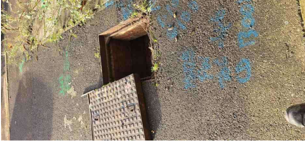
MH28X_e42b9812-bda0-4a33-aaa0-95b41106b23d_20241125_104542.jpg, 00:00:01, 0.00 m Start node, manhole, reference: MH28
