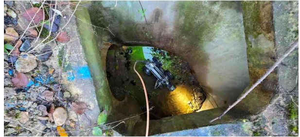
X_eef80fef-569a-412d-a87a-84c72ef6bb35_20241125_144828.jpg, 00:00:01, 0.00 m Start node, manhole, reference: MH92
