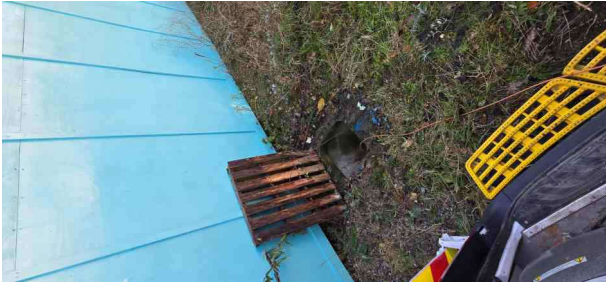
X_2586be45-4d85-47f3-9d48-08431449bb65_20241125_144824.jpg, 00:00:01, 0.00 m Start node, manhole, reference: MH92
