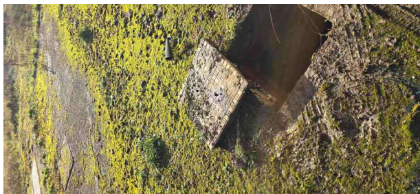
MH50X_f7da4275-0fb1-49b8-89da-72c9da125b0b_20241125_123421.jpg, 00:00:01, 0.00 m Start node, manhole, reference: MH50
