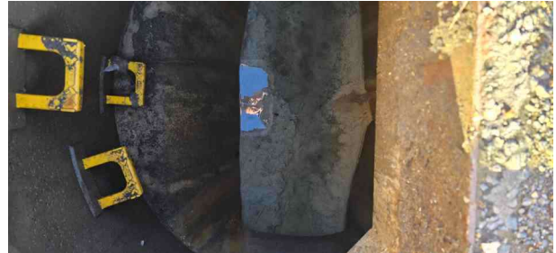
MH61X_449bec40-dc47-42f4-b402-821d3b46e9b5_20241125_135540.jpg, 00:00:01, 0.00 m Start node, manhole, reference: MH52
