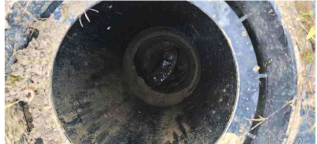
MH70X_16ffa554-662e-4a19-806b-834db8797b30_20241125_142815.jpg, 00:00:01, 0.00 m Start node, manhole, reference: MH70
