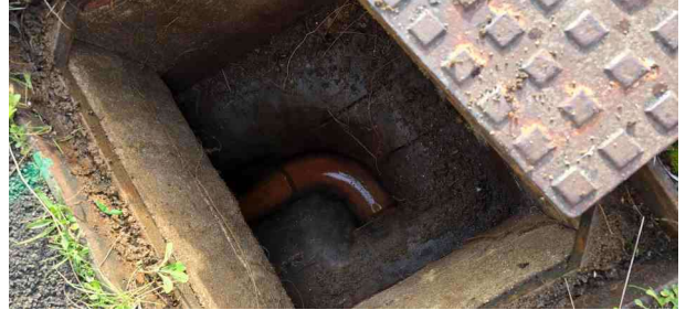
MH32X_9cfc2b80-a715-4459-88b9-deff1fcf4eab_20241125_105303.jpg, 00:00:01, 0.00 m Start node, manhole, reference: MH31
