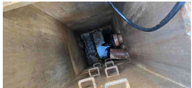
MH70X_482b3a68-3968-4f9b-934f-2755644c4826_20241125_142839.jpg, 00:00:26, 0.50 m Finish node, manhole, reference: MH69
