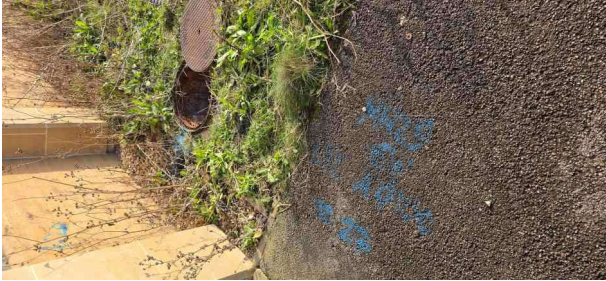
MH29X_175b347a-573a-4b10-8026-45d9110113f6_20241125_113020.jpg, 00:00:01, 0.00 m Start node, manhole, reference: MH29
