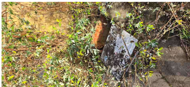
MH27X_576a0bc6-2da8-46f8-a3c9-27a2f49a2934_20241125_113251.jpg, 00:00:01, 0.00 m Start node, manhole, reference: MH27
