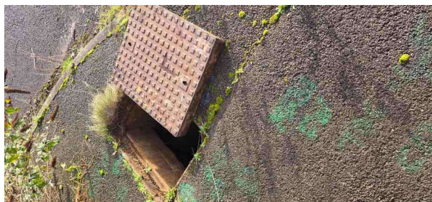
MH30X_36e63094-db5f-4636-ba2e-040563ca36ee_20241125_105029.jpg, 00:00:41, 6.18 m Finish node, manhole, reference: MH31
