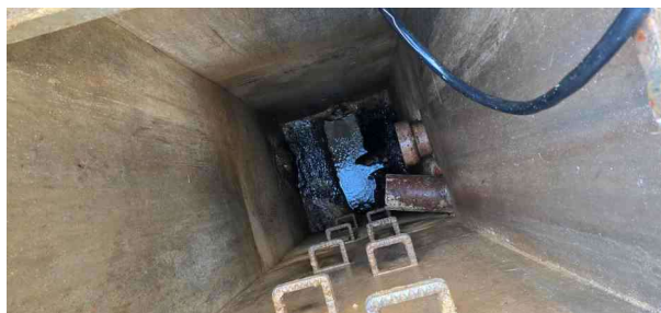
MH63X_fc3eee03-1a09-4fa9-a55e-c192e3ece00d_20241125_142804.jpg, 00:00:41, 7.64 m Finish node, manhole, reference: MH69
