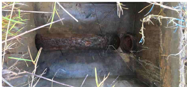
MH66X_2dc65504-d53d-443b-888b-a4185d0b8c0d_20241125_143058.jpg, 00:00:01, 0.00 m Start node, manhole, reference: MH66
