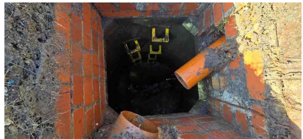
MH61X_95386cbb-045a-4908-ae61-5f8a9d181394_20241125_135443.jpg, 00:03:38, 32.41 m Finish node, manhole, reference: MH61
