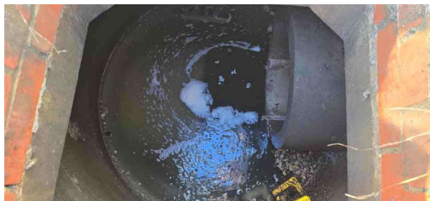
MH50X_3d1301d5-ca3e-409b-a436-1ac2832fe5e6_20241125_123435.jpg, 00:00:01, 0.00 m Start node, manhole, reference: MH50
