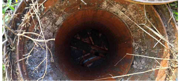
MH29X_900c1148-395f-4970-9e14-bc5ba8ed2804_20241125_113025.jpg, 00:00:01, 0.00 m Start node, manhole, reference: MH29
