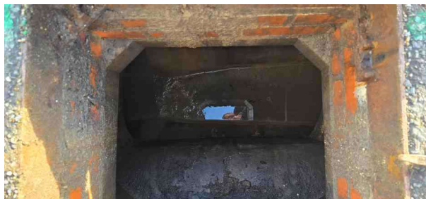
MH52X_db8eb618-e844-4224-9c42-6bb9f034aebd_20241125_115553.jpg, 00:00:01, 0.00 m Start node, manhole, reference: MH33
