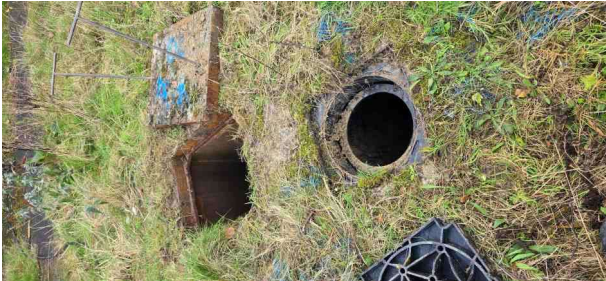
MH70X_952ce354-e7cf-4cab-a660-69bb7fe629e2_20241125_142811.jpg, 00:00:01, 0.00 m Start node, manhole, reference: MH70
