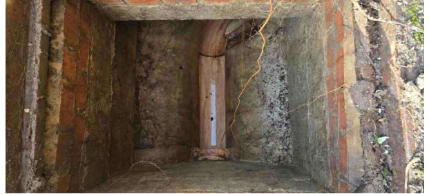
MH28X_122d1d2b-3703-4886-af15-0fd485a07d1e_20241125_104619.jpg, 00:00:01, 0.00 m Start node, manhole, reference: MH28
