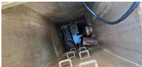
MH64X_b008573f-6747-4f00-aa6c-8ff2cf7564c6_20241125_142612.jpg, 00:00:50, 12.02 m Finish node, manhole, reference: MH69
