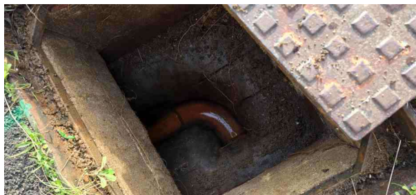
MH31X_692cda61-f981-4fc9-8050-62c47045bd7c_20241125_104641.jpg, 00:00:01, 0.00 m Start node, manhole, reference: MH31
