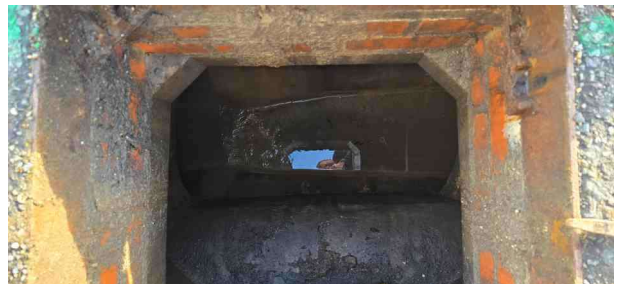
MH33X_115bf01f-265c-4dc9-b4e9-34a2b1cad7e3_20241125_145344.jpg, 00:03:02, 29.66 m Finish node, manhole, reference: MH33
