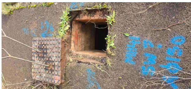
MH31X_ebb73134-f690-408e-8e0d-5e6dd5cd9f5c_20241125_104914.jpg, 00:01:07, 14.10 m Finish node, manhole, reference: MH41
