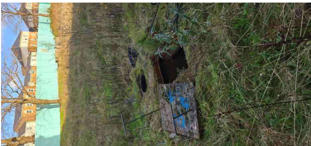
MH70X_70be9e61-a083-4eb8-9561-a24162f15128_20241125_142836.jpg, 00:00:26, 0.50 m Finish node, manhole, reference: MH69
