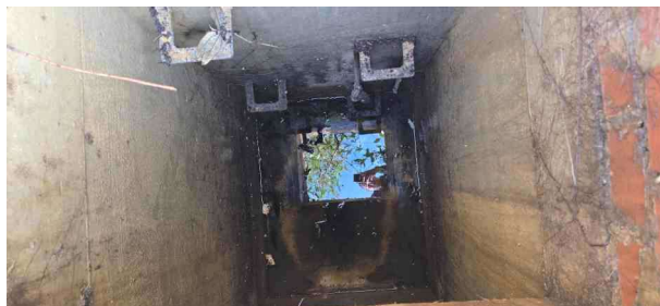
MH27X_fe3962d4-d31e-4d1b-9c03-24360ed70b05_20241125_113255.jpg, 00:00:01, 0.00 m Start node, manhole, reference: MH27
