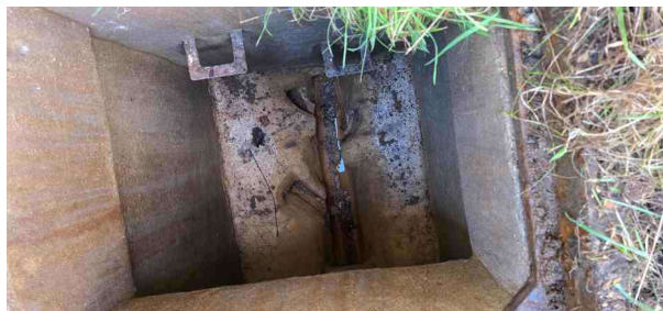
MH63X_f4076f48-0765-4e20-82e3-76d467fc6afd_20241125_142655.jpg, 00:00:01, 0.00 m Start node, manhole, reference: MH63
