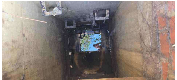
MH29X_d4099cf8-2af2-4cb6-8f57-635ec8cf874a_20241125_113040.jpg, 00:00:47, 7.64 m Finish node, manhole, reference: MH27
