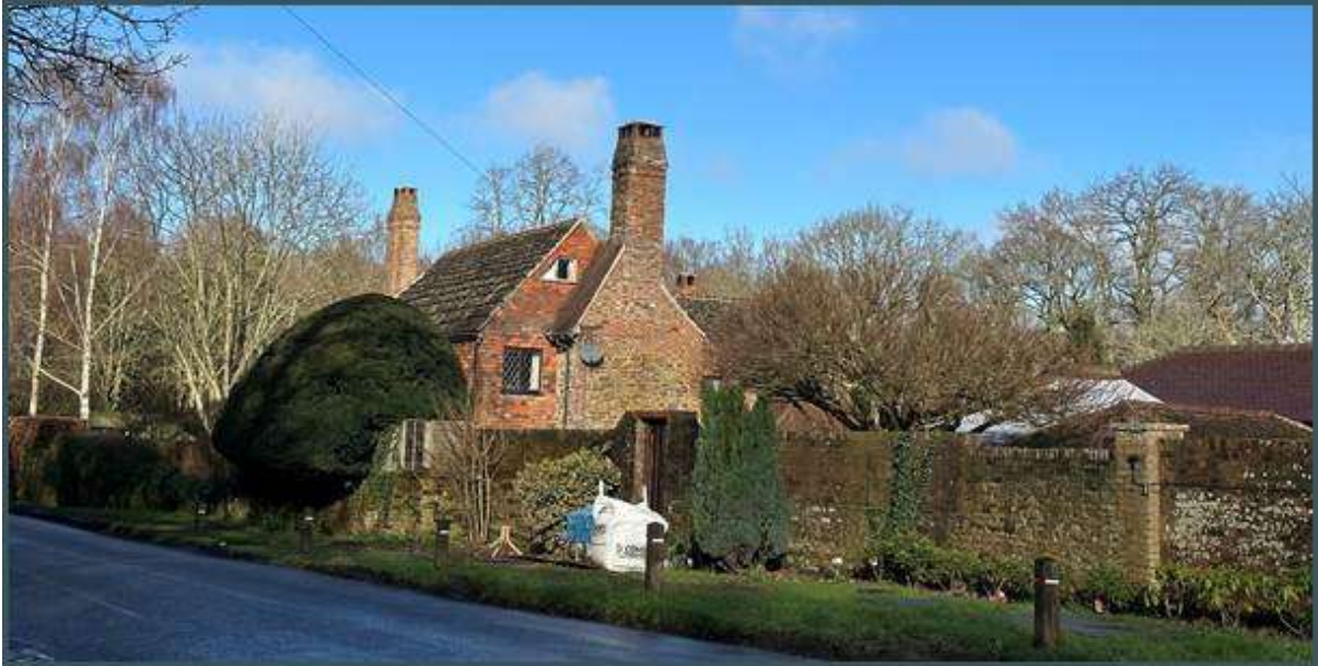
Above: the Grade II listed Kings Farmhouse is 65m to the north of the proposed warehouse.
