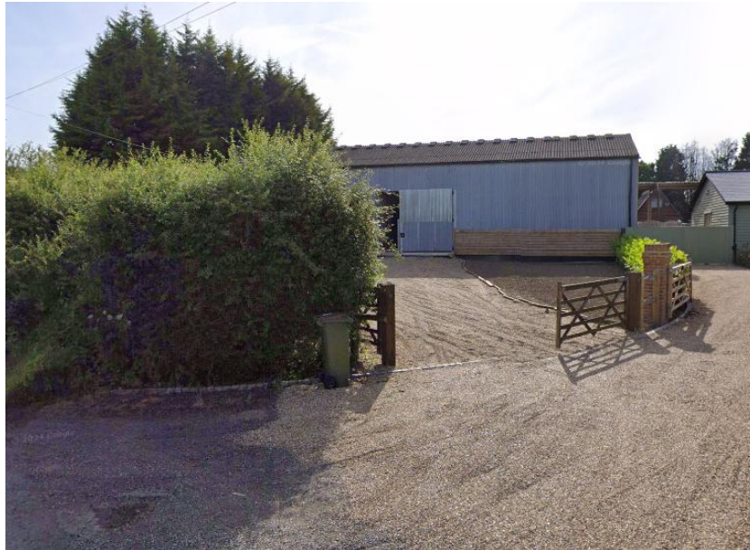
Image 1: Site viewed from Sincox Lane (June 2024)
