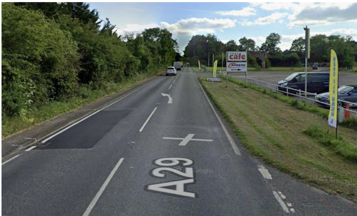
Figure 5: Stane Street looking south (with road gully on east side of the highway)
