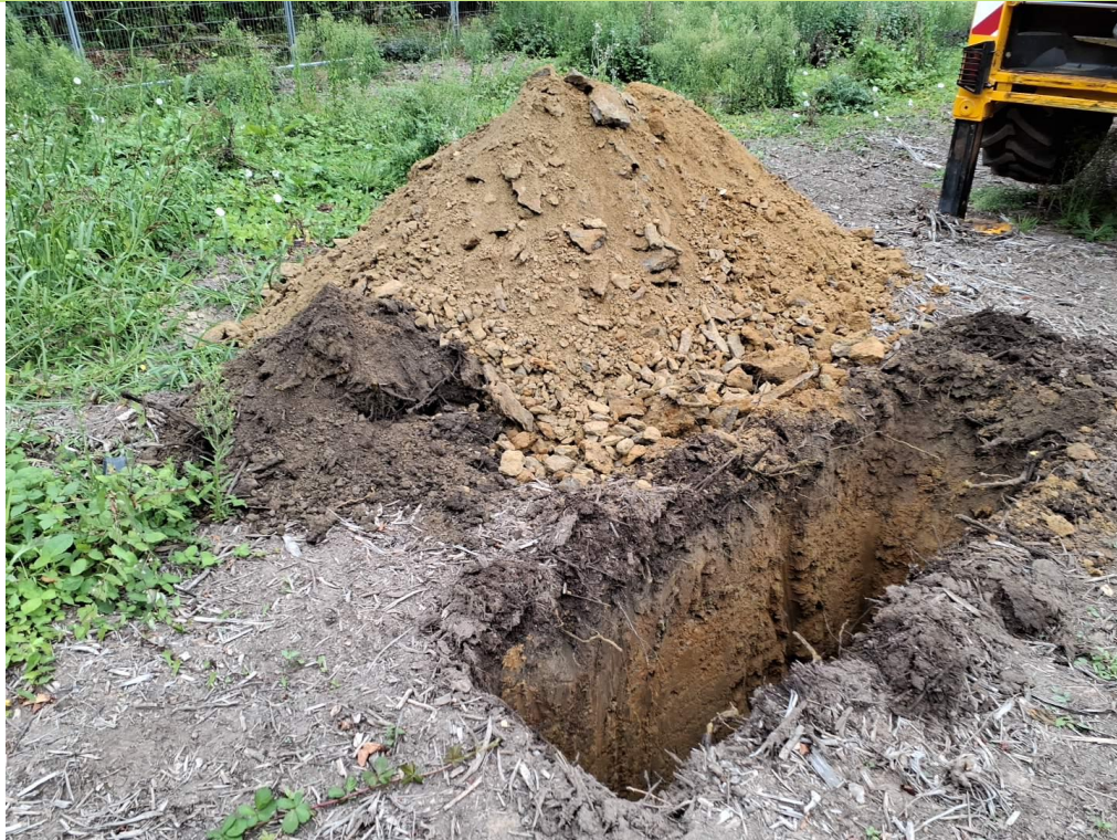
Plate 21 – Overview of topsoil and Hythe Formation from TP402
