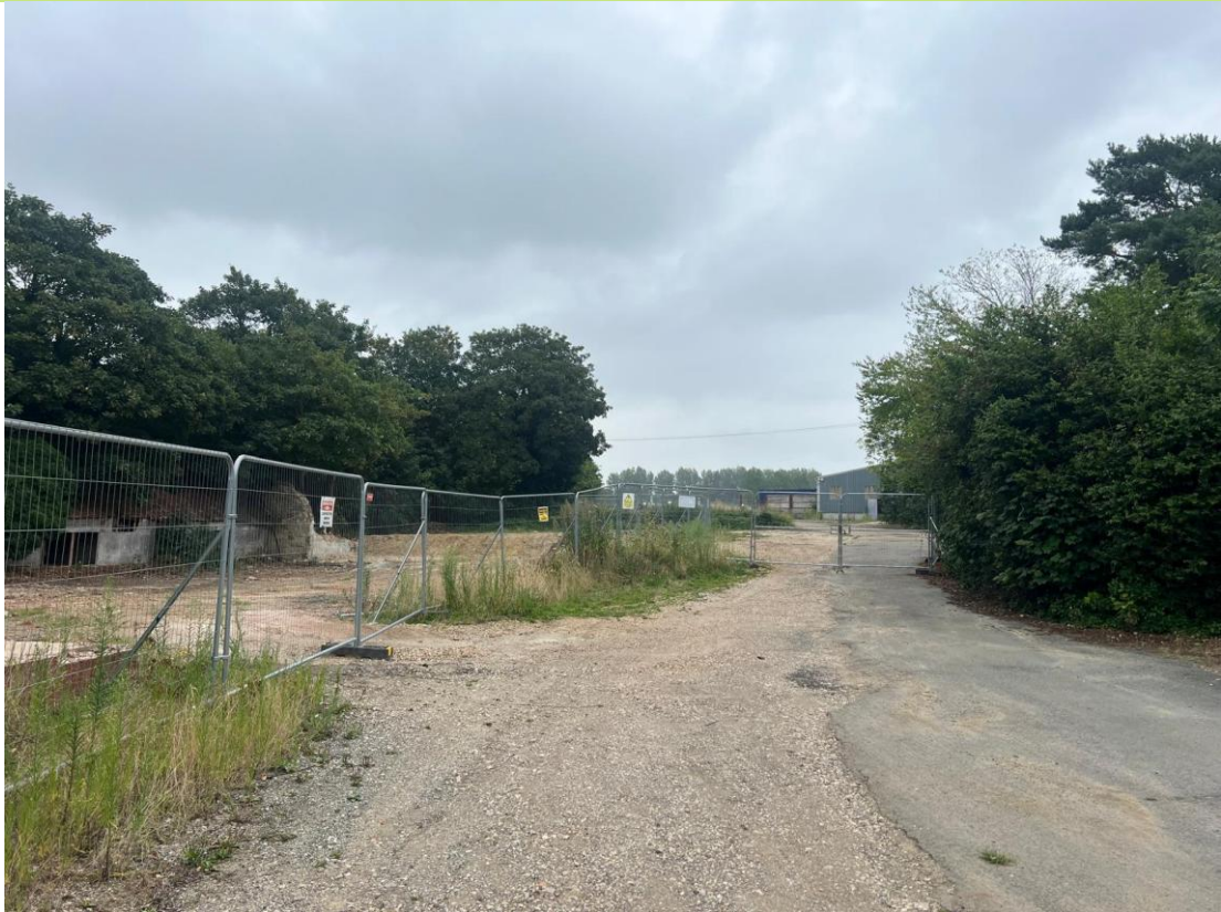
Plate 1 – Facing east, main site entrance. Empty workshop unit visible front right. Cleared area after demolition works left.
