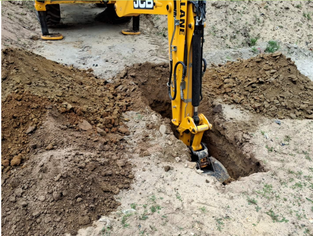
Plate 19 – Overview of trial pitting TP401 with JCB 3CX.
