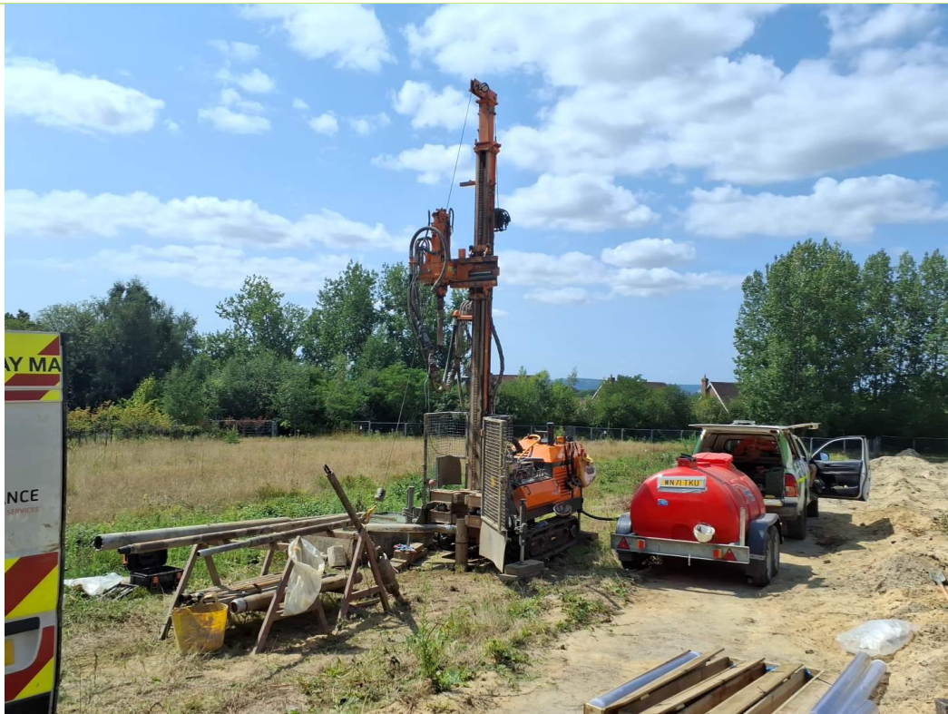
Plate 10 – Overview of drilling rotary core borehole BH401.
