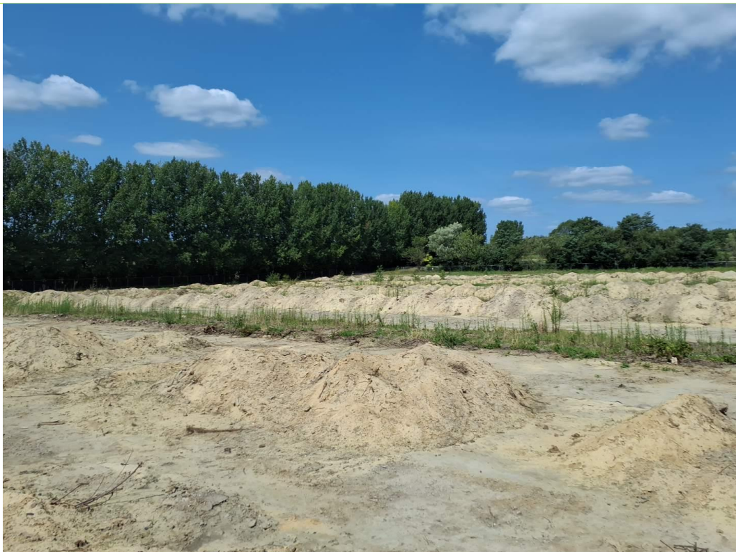
Plate 12 – Overview of southeastern region of the site where polytunnels were previously present.
