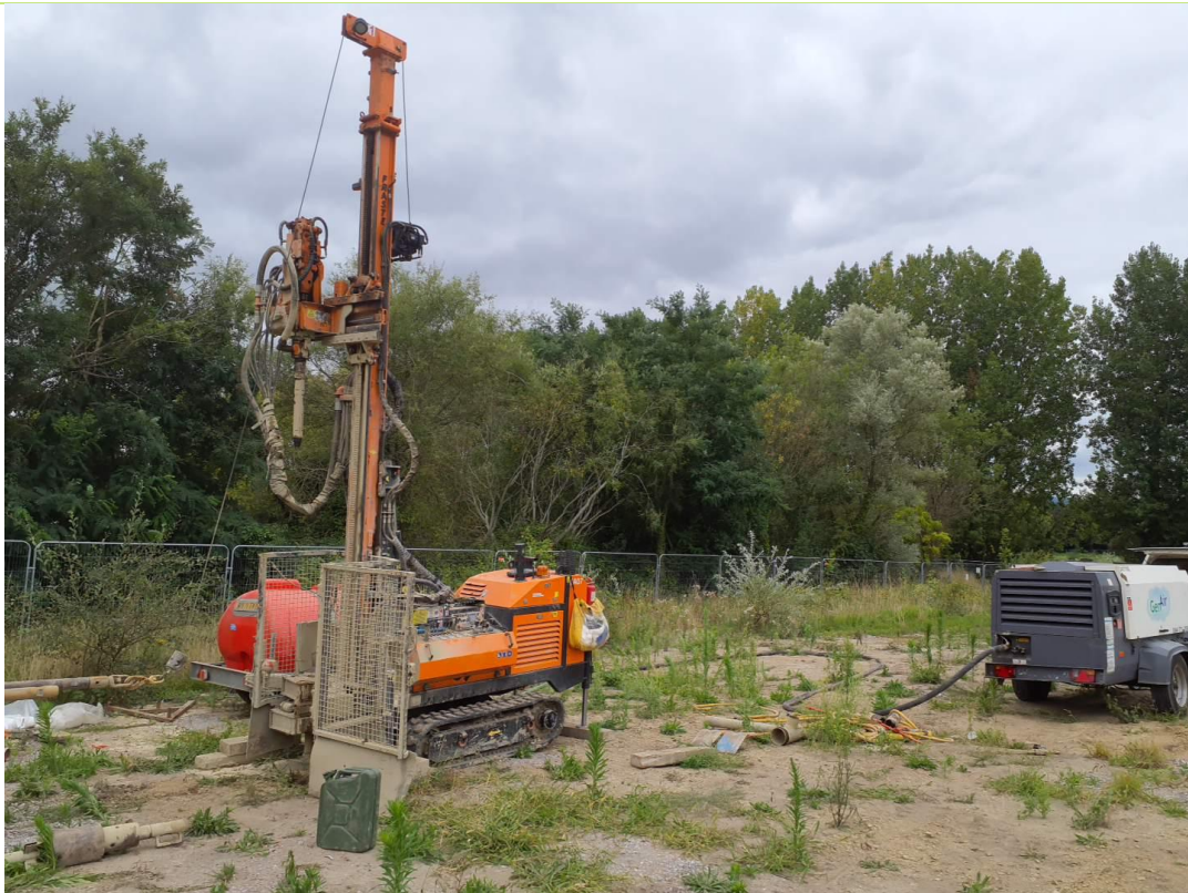
Plate 16 – Overview of BH404 being drilled using compressor.
