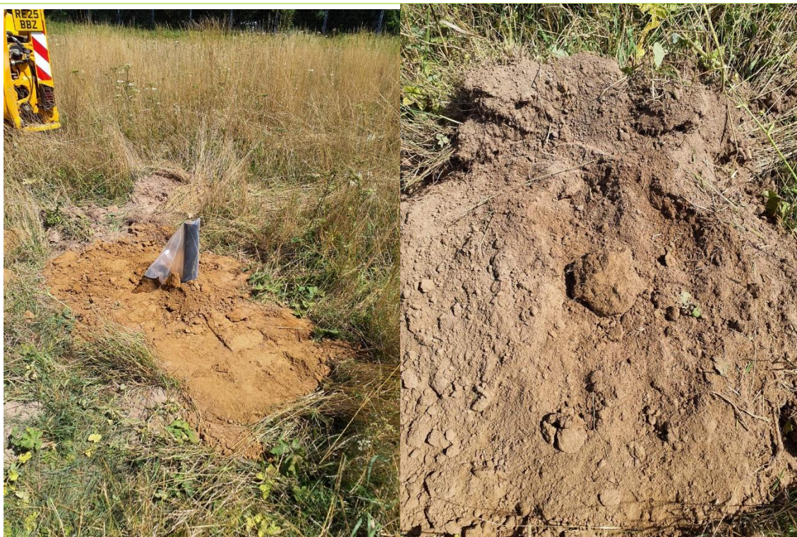
Plate 24 – SA403 installation (left) and recovered topsoil (right)
