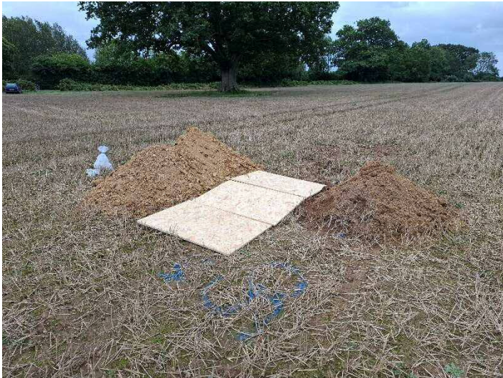
Photograph 11 – A view of a soakaway pit being protected and made safe overnight.
