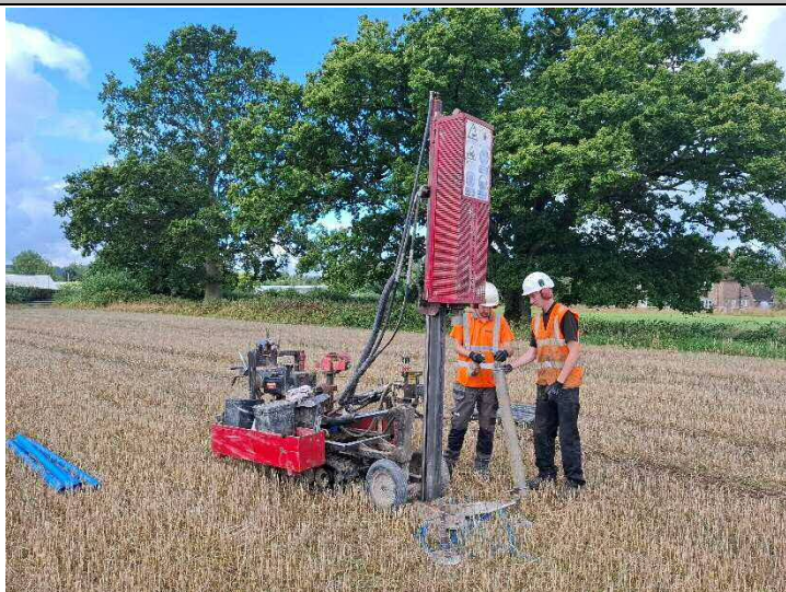
Photograph 3 – A view of a window sampling rig on position.
