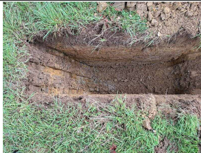
Photograph 8 – A typical view of a trial pit on site with stable sides throughout.
