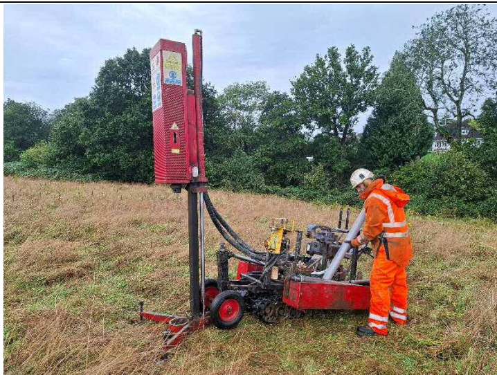
Photograph 5 – A view of a window sampling rig on position.
