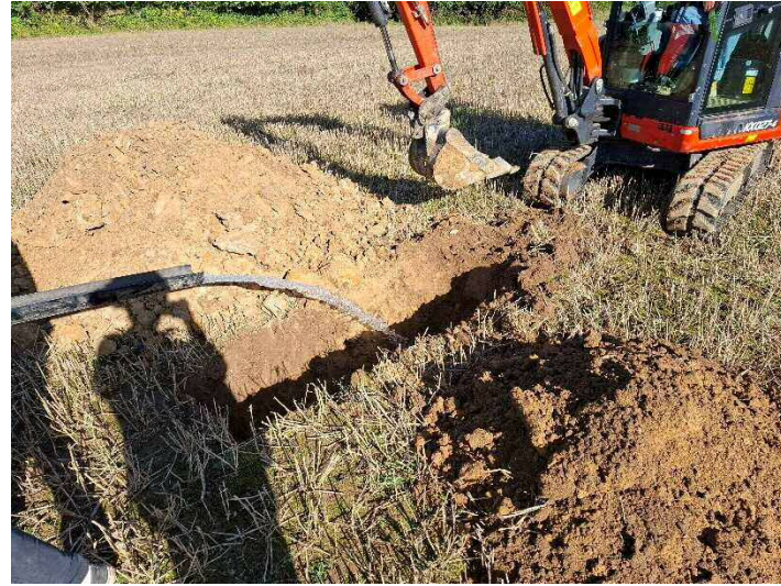
Photograph 10 – A view of a soakaway test being commenced on site.
