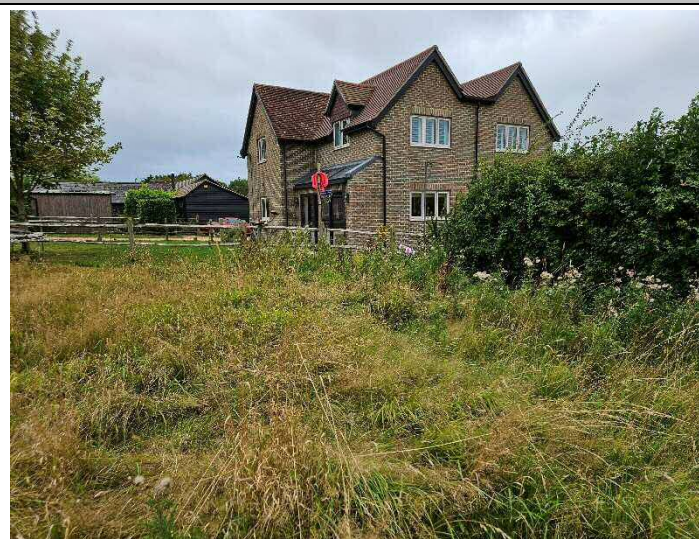
Photograph 4 – A view of the westernmost dwelling to the south of the site.
