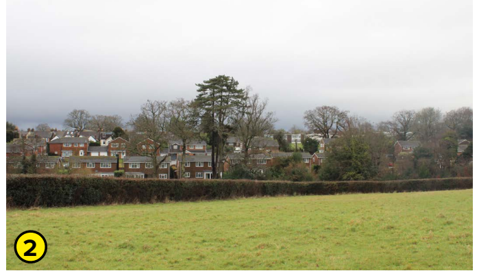
Photograph 2 – View looking north west towards existing houses to north of site.
