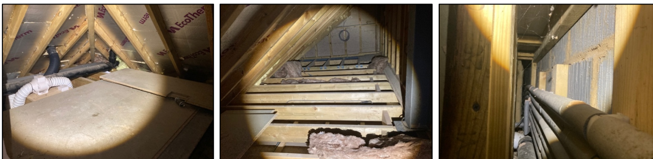
Photograph 2a, 2b & 2c. Views of Void 2, including an access section on the western elevation where the droppings were found (left), the largest section of the void (centre) and the end section of the void that was obstructed by piping and could not be fully explored (right).
