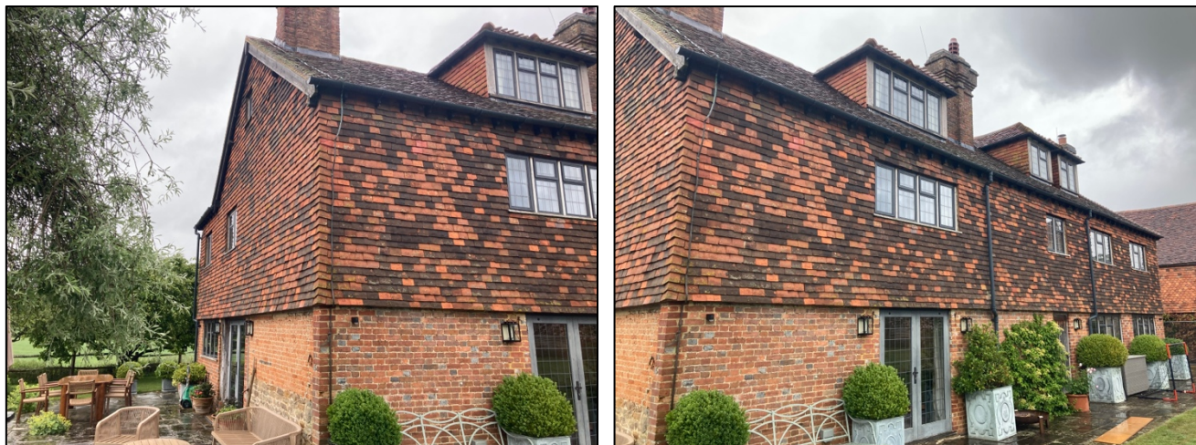
Photograph 3a & 3b. The western (left) and southern (right) elevations of the main dwelling at Town House Farm. Two droppings belonging to a Natterer's bat were identified under hanging tiles in the south-west corner.
