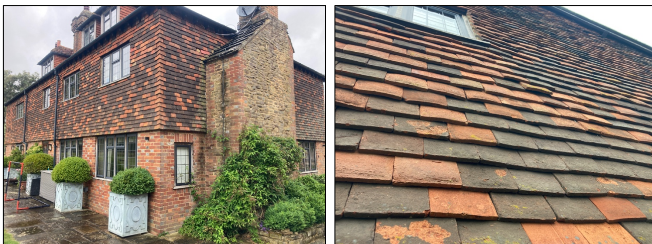
Photograph 4a & 4b. The eastern elevation of Town House Farm, with examples of suitable bat roost features through gaps under hanging tiles that are present across all elevations of the property.
