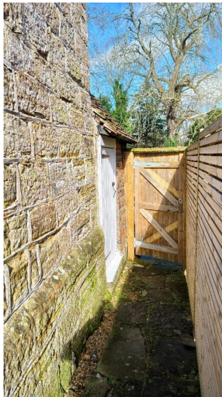
Fig.12 Photos of the existing east side of the garden and boundary
