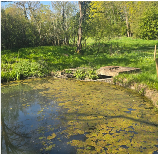
Location C – Pond Outfall to Culvert
