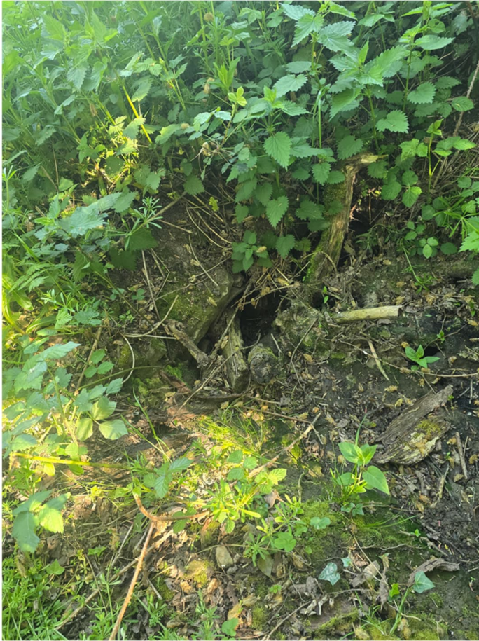
Location A - Culvert Crossing
