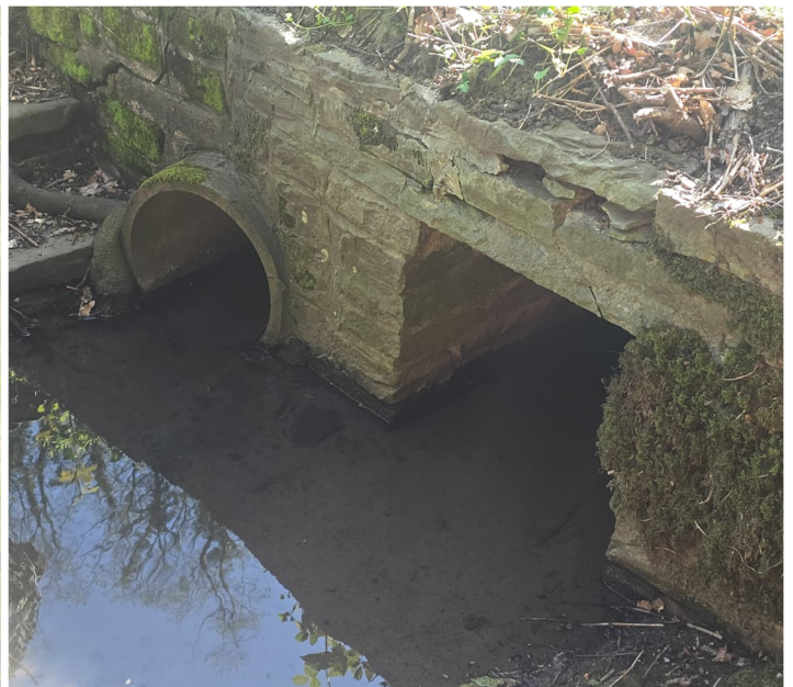
Location D – Culvert Outfall to Watercourse
