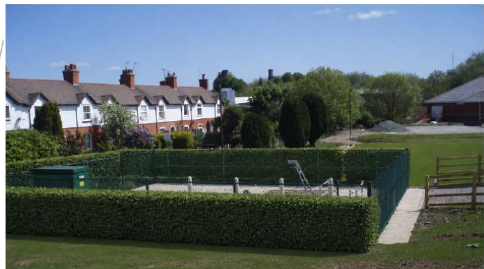
Example pumping station appearance.
