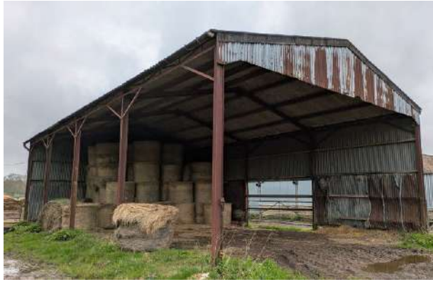
Photo 5: Northern and eastern elevations of B8.
