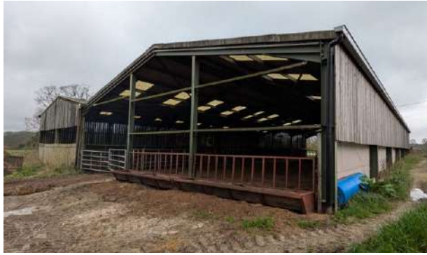
Photo 16: Southern elevation of B15.
