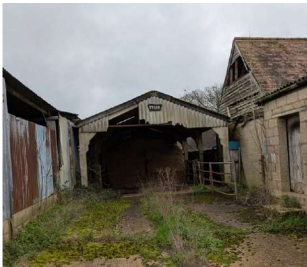
Photo 7: Northern elevation of B10 in centre of image, with eastern elevations of B12 and B11 in right side of photo and western elevation of B9 in left side of photo.
