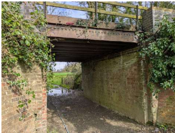
Photo 4: Southern elevation of B5.
