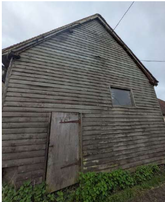
Photo 11: Western elevation of B12.
