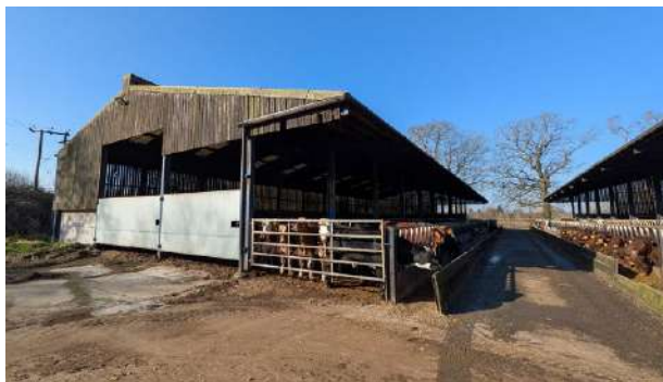
Photo 3: Northern and eastern elevations of B4 in the centre of the image, with southern elevation of B3 in right side of photo.
