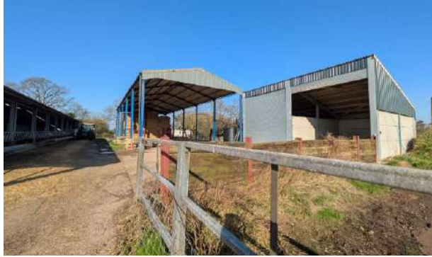
Photo 1: Southern and eastern elevations of B1 in the centre of the image, with northern elevation of B2 in left-side of photo and southern and eastern elevations of B16 in right side of photo.
