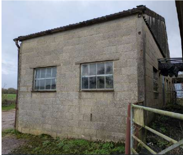
Photo 9: Southern and western elevations of B11.
