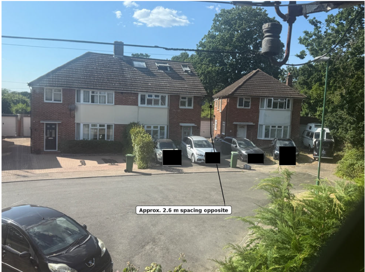
Figure 2: View directly opposite the proposed dwelling, illustrating the different roof forms and roof treatments within the immediate street scene.
