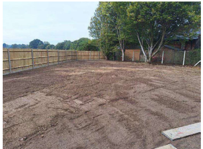
Plate 8: Plot 1 & 2 completed (STL 01.10.2025).
