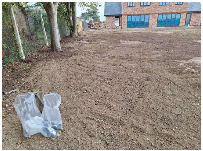
Plate 6: Southern part of Plot 1 completed (STL 01.10.2025).
