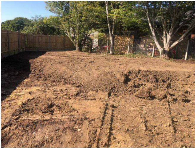
Plate 5: Photograph provided from site showing the placement of topsoil to the end of Plot 1.
