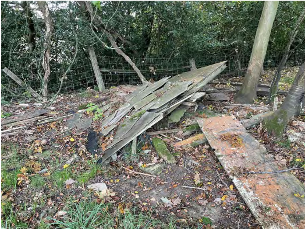
Photograph 1: View of stockpile 1, mainly potential asbestos containing material (old roofing sheets) within the southwestern area of the site.
