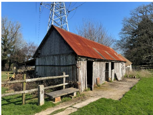
Photograph 1. The barn viewed from the south-west.
