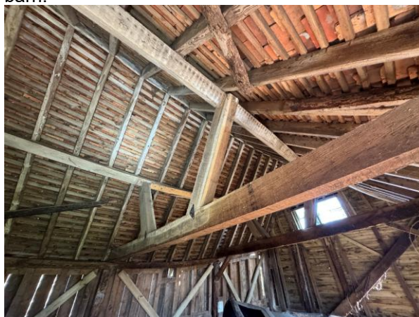
Photograph 4. Interior of the old section of the barn.
