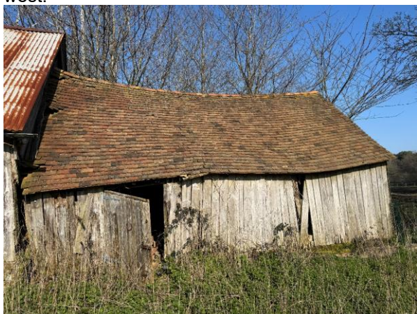
Photograph 3. The barn viewed from the south.
