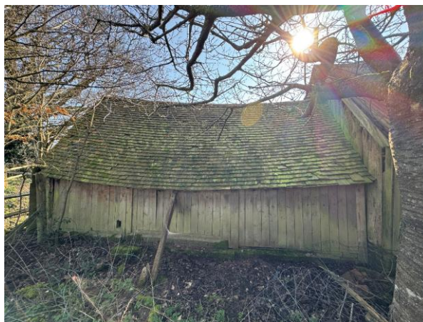
Photograph 8. The barn viewed from the north.
