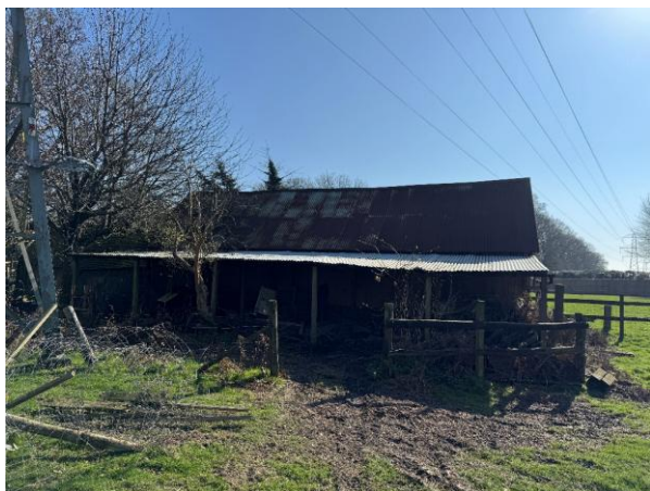
Photograph 7. The lean-to section of the barn.
