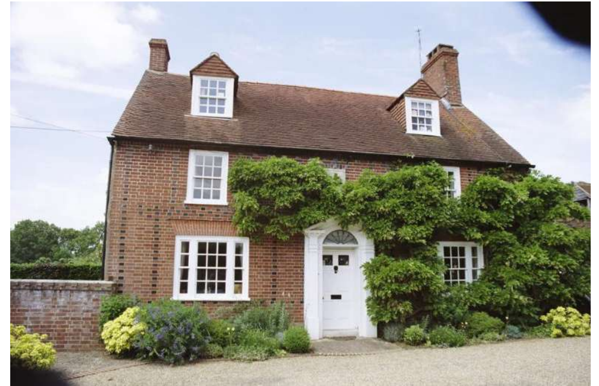
East elevation of Midway House (c) Historic England image
