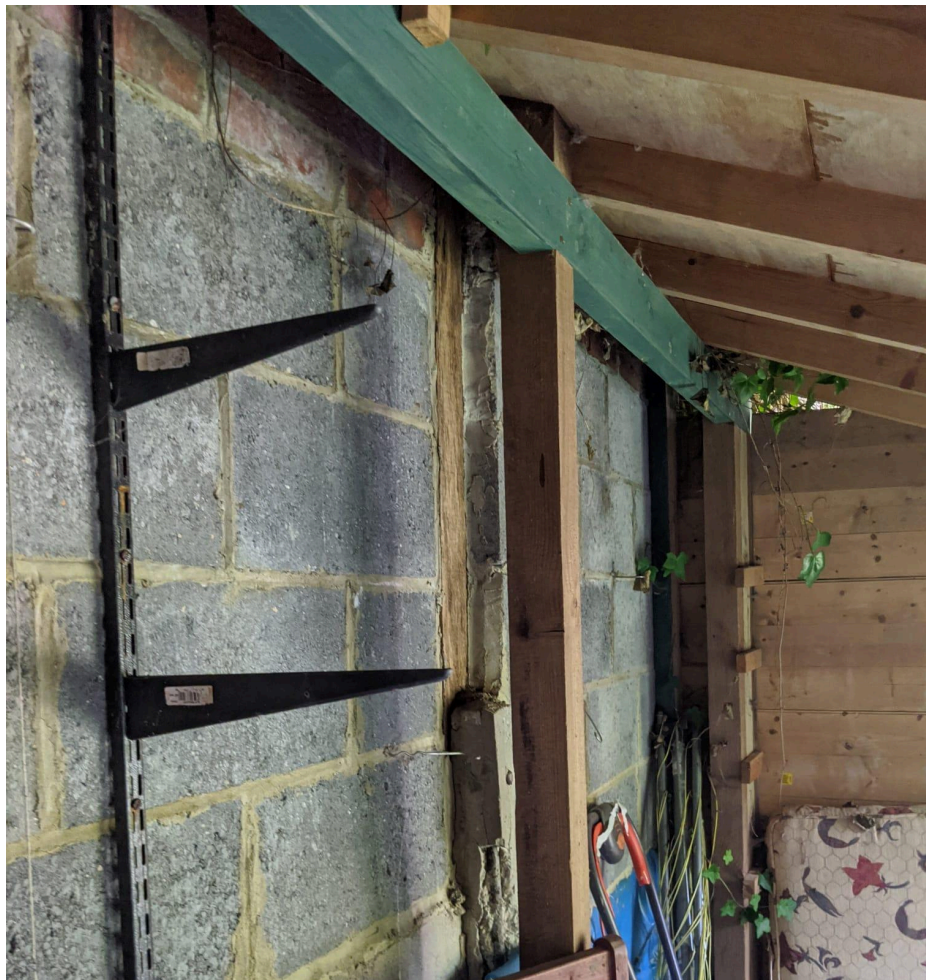
Image 2: Breeze block boundary wall to rear of existing shed
