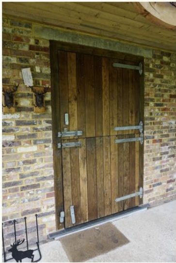
NEWBARN DOOR TO MATCH EXISTING BUILDING STYLE
