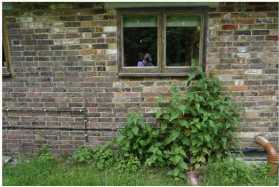
DATED BRICKWORK WITH NEW REPAIR
