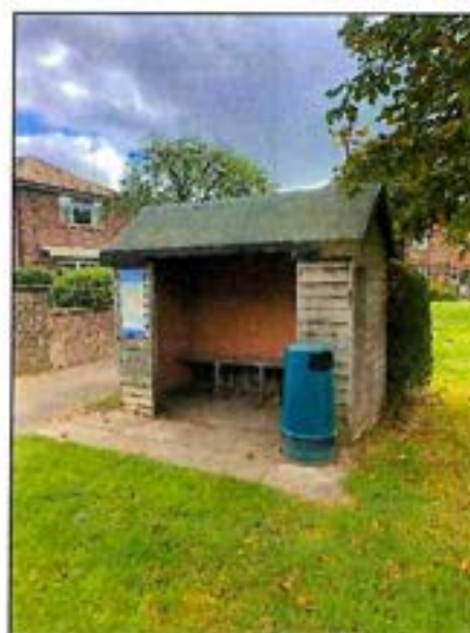
Photograph 5: Sheltered Bus Seating Area
