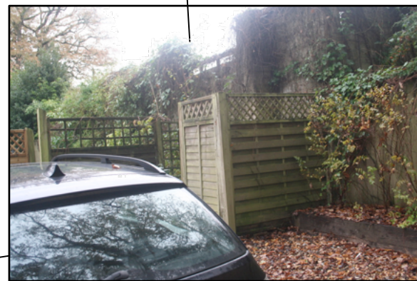
Boundary masonry wall, bin store and fencing
