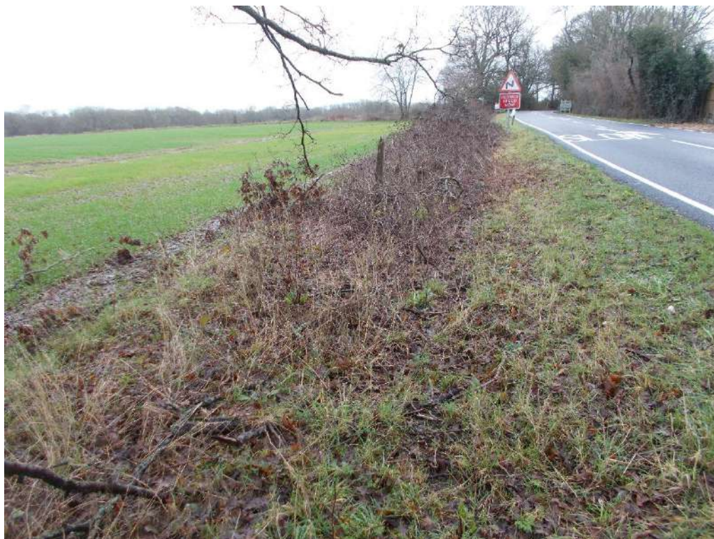
Photo 4: Degraded ditch in hedgerow on opposite side of Marches Road.
