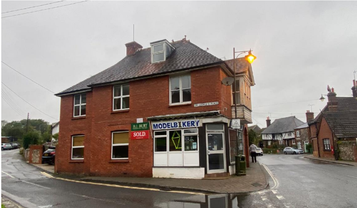
Fig 2. Existing view from the High Street ( Courtesy of DAS )
