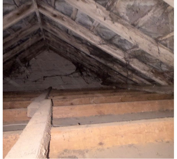
Plate 8: Northern Roof Void Section
