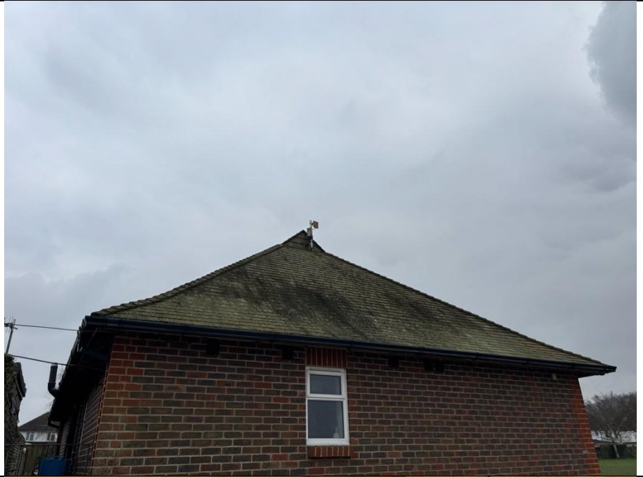
Photograph 6: Tiled roof on changing rooms
