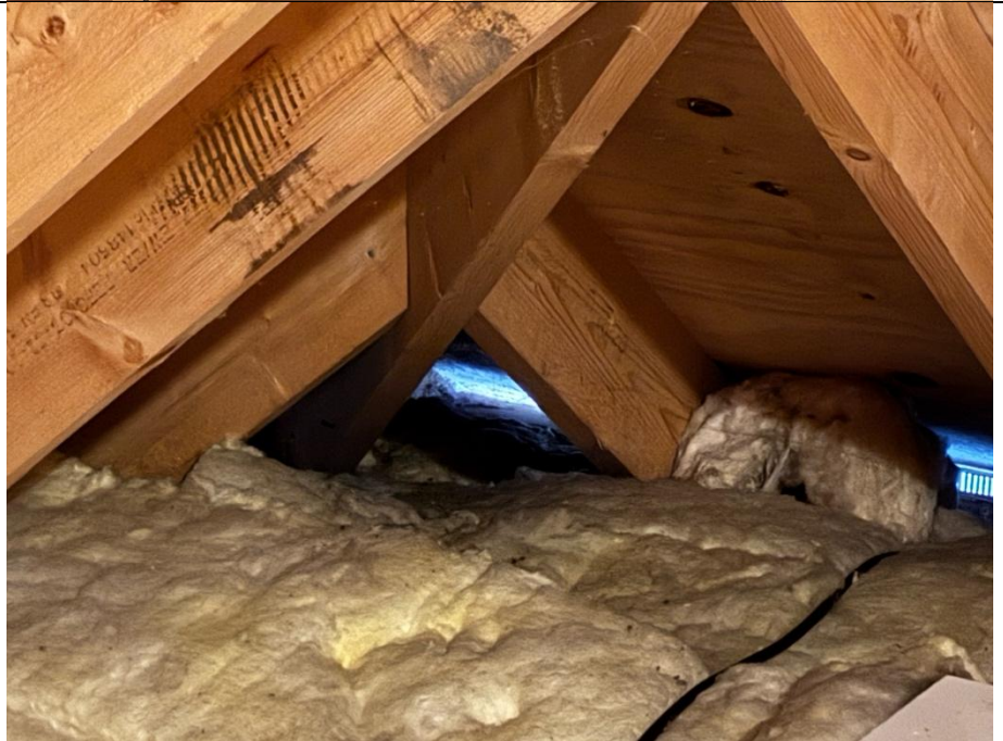
Photograph 9: Corner of loft void
