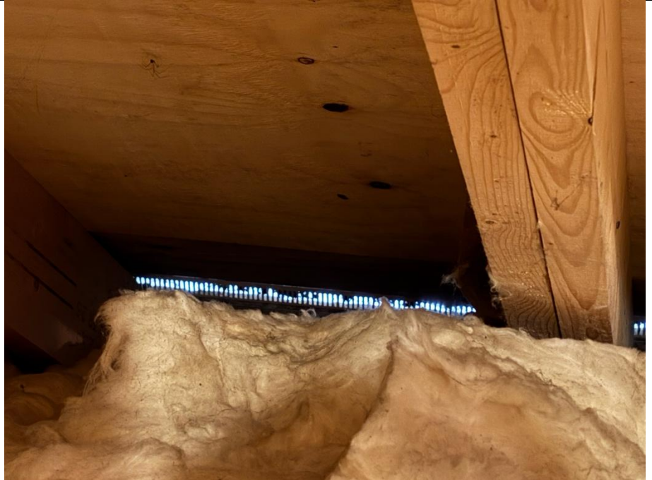
Photograph 7: Example of grate present in loft void around 90% of the eaves.
