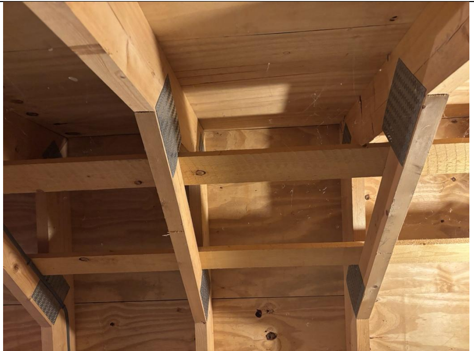
Photograph 8: Changing room loft void internal
