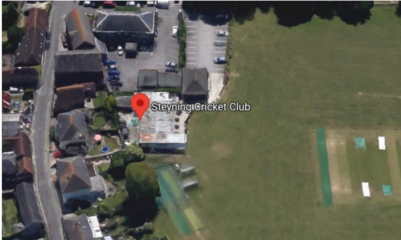
2.7 Site looking South (Source: Google Maps)
