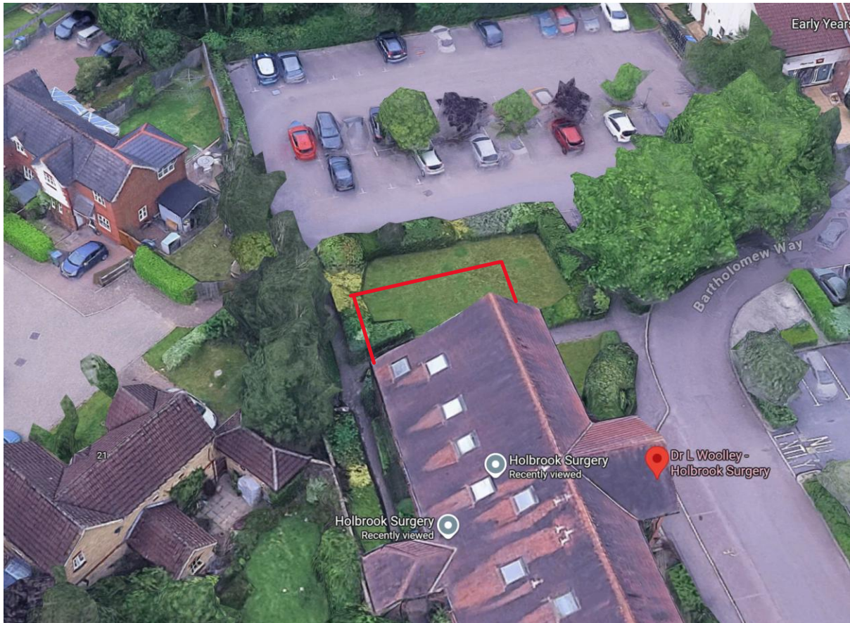
Photo 11 - Google Image showing context view from South – Note 20 Highdown View first floor window positions indicated but heavily screened by trees and planting ©Google
