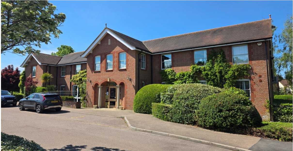
Photo 1 – Front (East) Elevation
