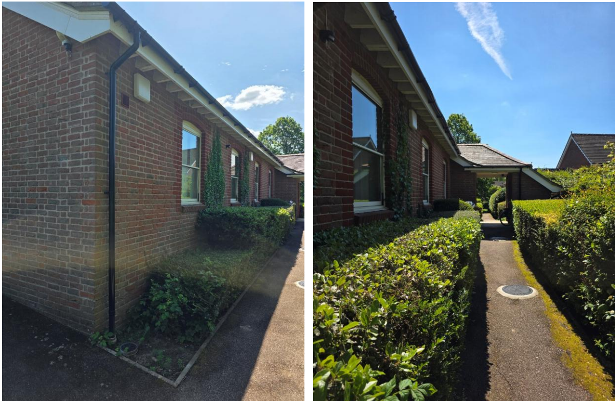
Photo 4/5 – Rear (West) elevation. Whole elevation cannot be photographed due to site constraints and location of boundary
