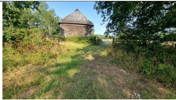
Plate 3. Access leading to Barn
