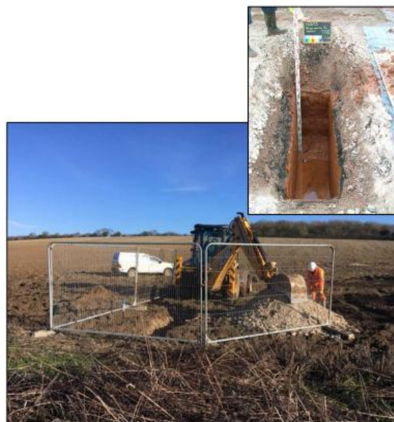
Figure 4 - Example Test Pitting
