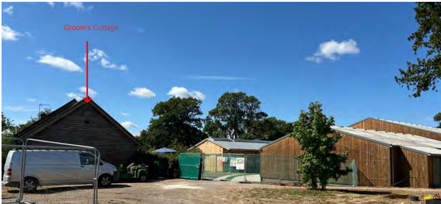
Approaching the Groom's Cottage from the driveway with the Poolhouse and Large Sheds under construction to the right
