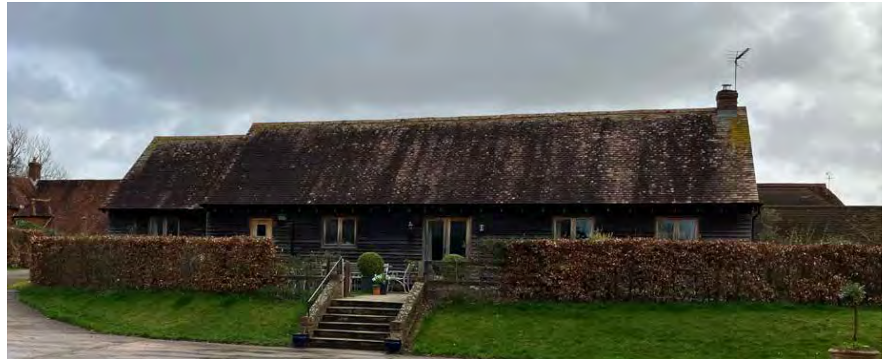
View of the Groom's Cottage from the west
