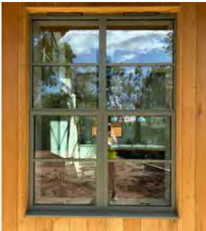
Metal framed windows to Poolhouse
