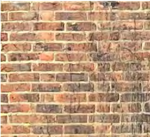
New brickwork to match existing
