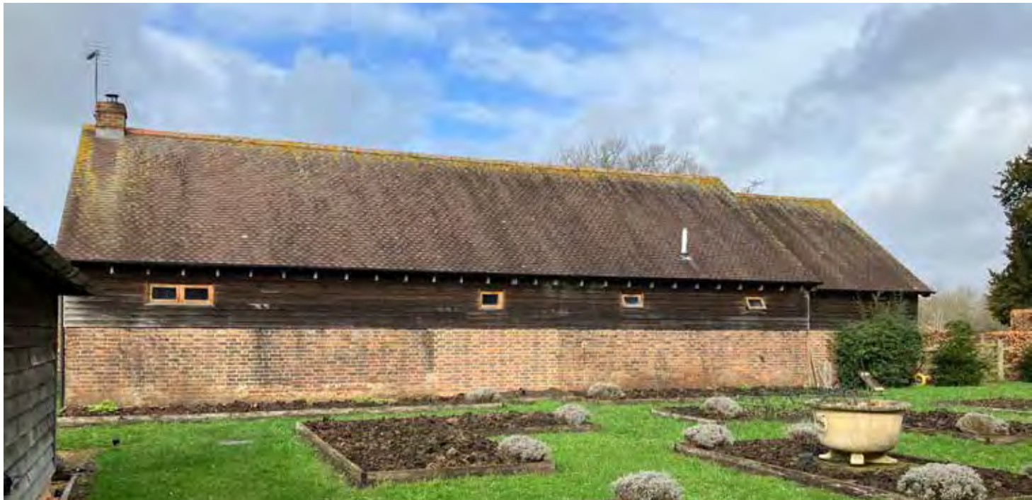
East elevation - an old opening is apparent from the newer brickwork
