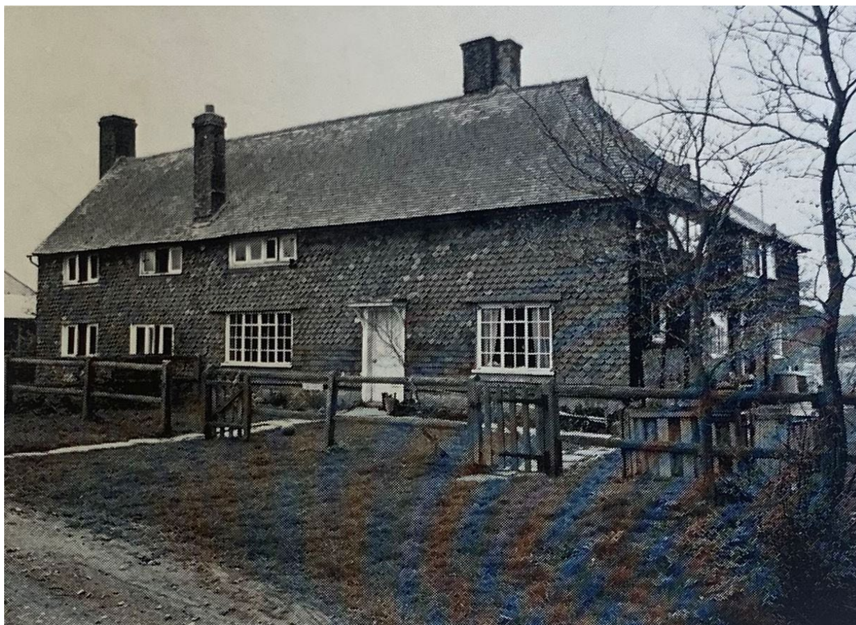
2.7 1969 photograph of the east and north elevations of the farmhouse, showing the former annexe at the northern end (West Sussex Records Office)
