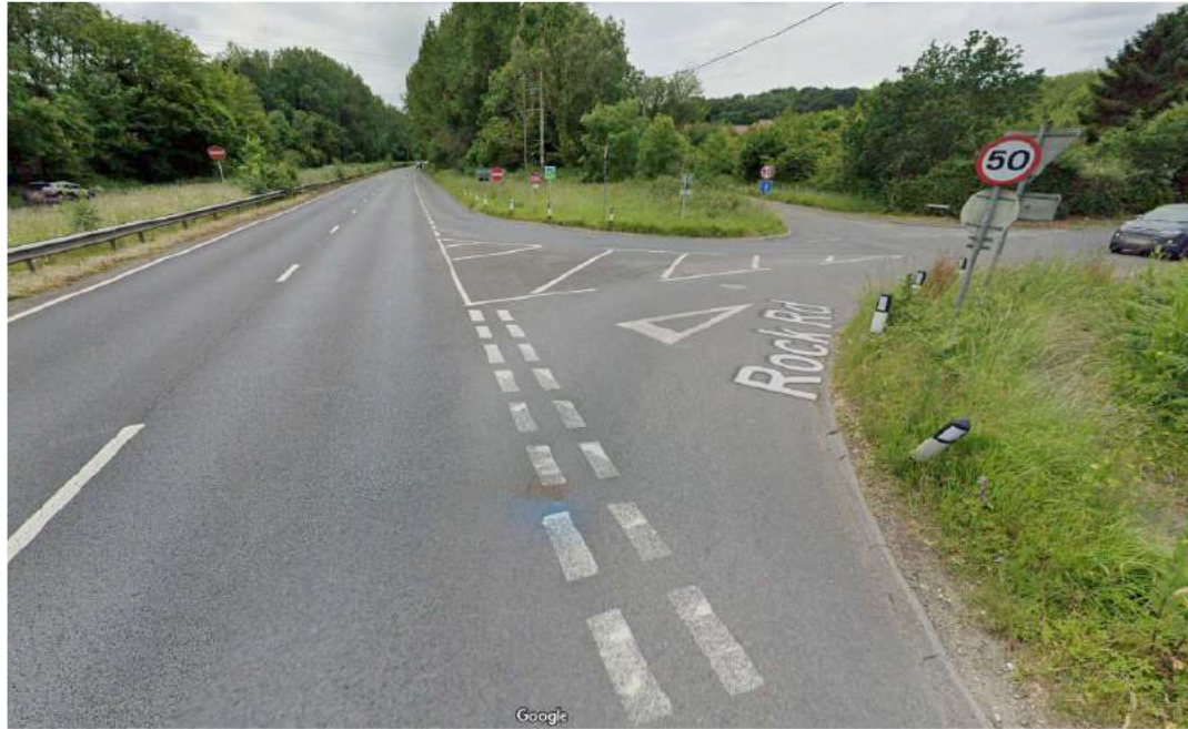
Figure 4-3 Photograph – Rock Road / A24
