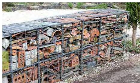
Retaining Gabion walls potentially filled with on site demolition waste
