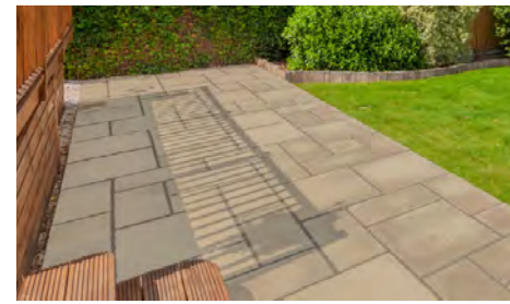
Terraces - Concrete Flag Paving
