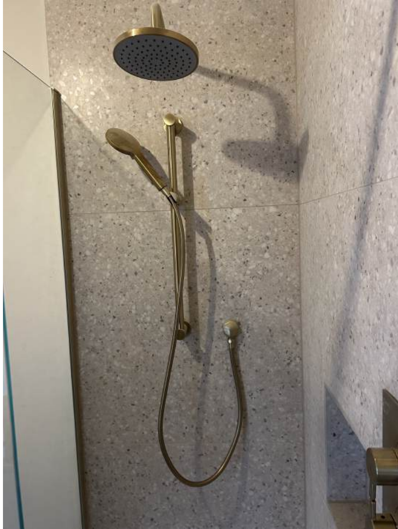
Thermostatic Shower Controls – Photo 4 Flow-regulated thermostatic mixer
