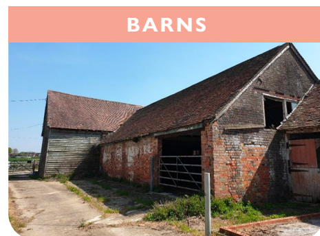
Existing historic barn
