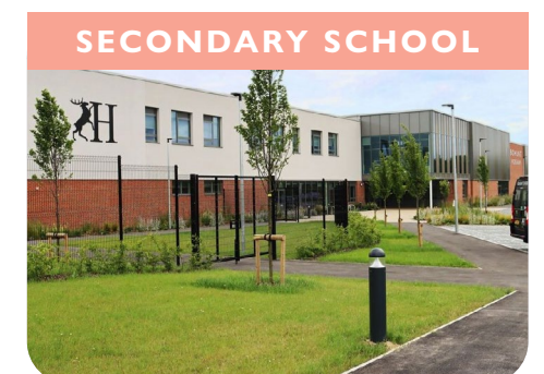
Bohunt School, North Horsham (Mowbray development)
