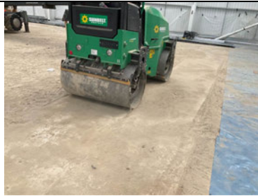
Substrate being rolled in preparation of gas barrier.
