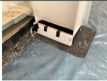
Restricted inspection to steel stanchions.
