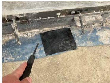
Probe testing to patched repaired armoured joint pin holes.
