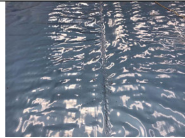
A typical hand welded membrane lap.
