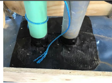
Typical double pipe penetration detailing.
