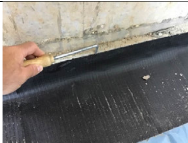
Probe testing the retro fit detailing to the base of the concrete stairs.
