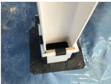
A restricted inspection took place of the steel stanchions due to miothene being in place at the time of our inspection.
