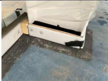
Restricted inspection to steel stanchion detailing.
