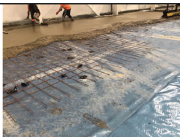
Overview of the membrane installation as the pour progresses.
