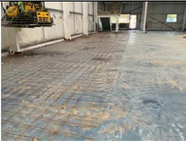
Overview of the Juta GP5 Gas Barrier installation.
