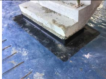
Overview of the detailing to the base of the concrete stair core.
