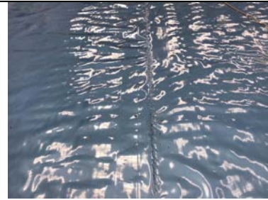
A typical hand welded membrane lap.
