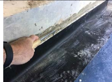
Probe testing all retro fit detailing.
