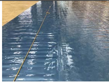
Overview of a hand welded membrane lap.
