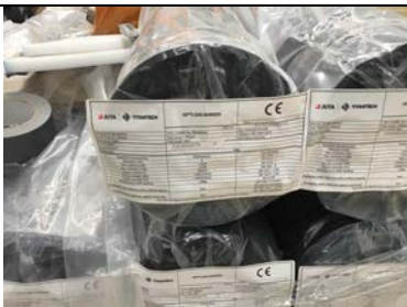
Evidence of the Juta GP5 gas membrane that has been installed on this project.
