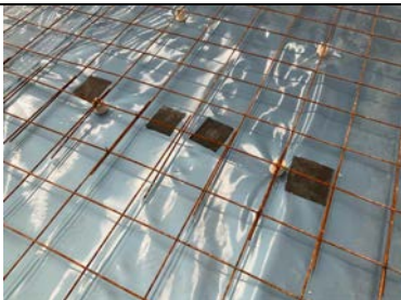
Installers own CQA patch repairs using Juta GP1 SAM.
