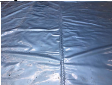
A typical auto welded membrane lap.
