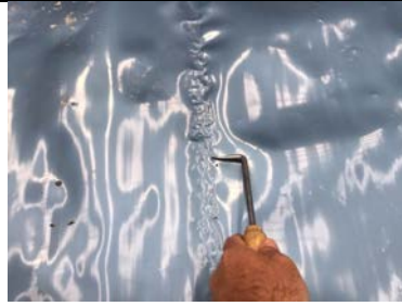
Probe testing a hand welded membrane lap.
