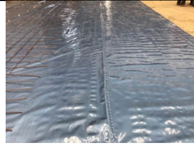
Overview of a auto welded membrane lap.
