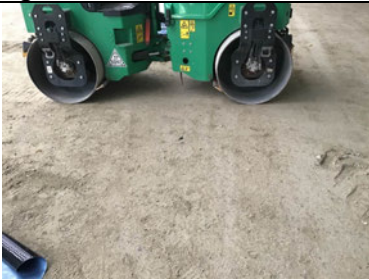
Evidence of the well rolled fine aggregate substrate that the membrane is being laid upon during the installation.
