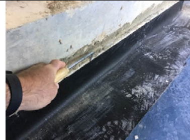
Probe testing all retro fit detailing.
