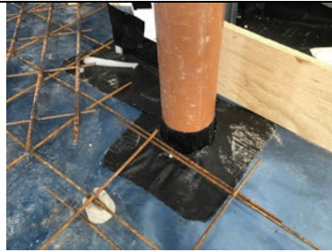
Typical pipe penetration detailing.
