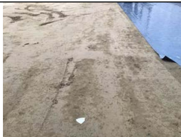
Evidence of the well rolled substrate prior to the membrane being installed.
