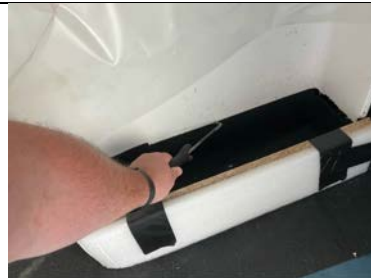
Probe testing to restricted steel stanchion.
