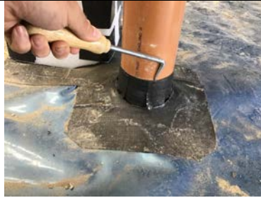
Probe testing a typical pipe penetration detail.
