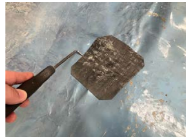
Probe testing to installers own CQA patch repair.
