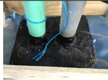
Typical double pipe penetration detailing.
