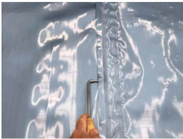
Probe testing all auto welded membrane laps.
