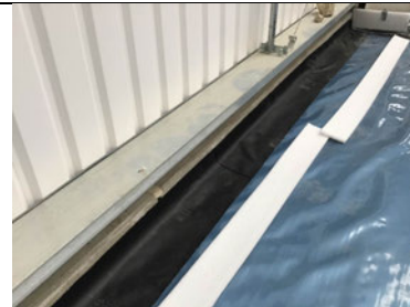
Overview of the perimeter termination detailing to the concrete curb stone.
