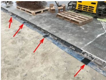
Armoured joint pin holes were patched repaired by installer using Juta GP1 SAM.
