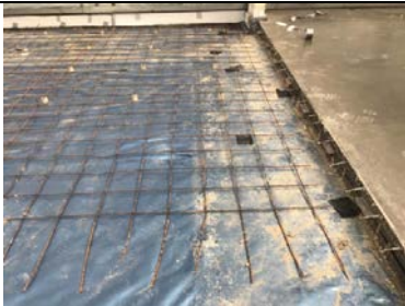
CQA repairs using Juta GP1 SAM to the pin hole damage along the armoured joint.
