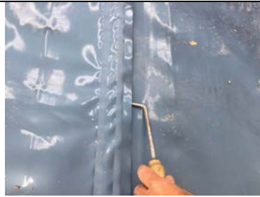
Probe testing an auto welded membrane lap.
