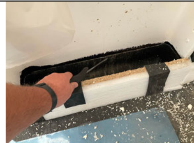
Probe testing to steel stanchion were possible.
