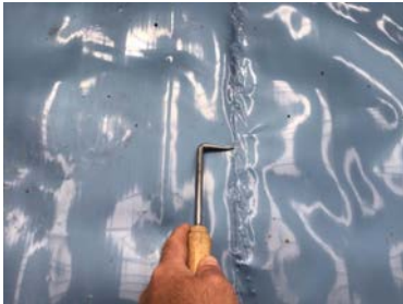
Probe testing all hand welded membrane laps.
