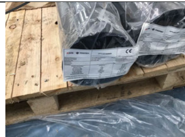
Evidence of the Juta GP5 Gas Membrane that has been used on this project.
