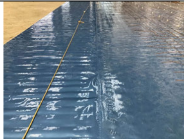
Overview of a hand welded membrane lap.
