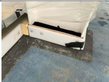
Restricted inspection to steel stanchion detailing.
