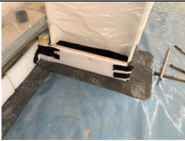
Restricted inspection to steel stanchion details.
