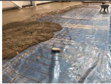
Overview of the membrane being installed on a just in time basis.
