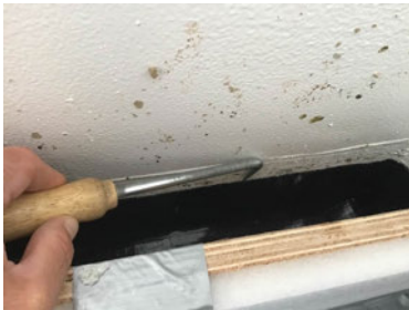
Probe testing a steel stanchion detail.
