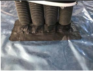
Typical pipe penetration detailing in unit 2 communal area.
