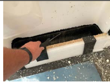
Probe testing to steel stanchion were possible.
