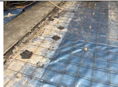
UK Membranes carried out their own CQA repairs as the pour progressed.
