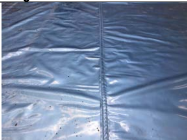
A typical auto welded membrane lap.
