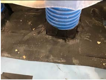
Typical pipe penetration detailing.
