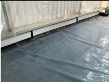
Restricted inspection of the retrofit termination detailing to the perimeter cladding rail.
