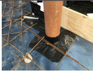
Typical pipe penetration detailing.
