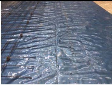
Overview of a hand welded membrane lap.
