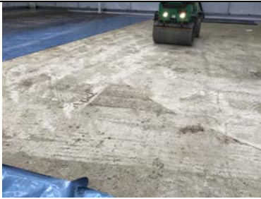
Evidence of the rolling machine used on the sand blinded substrate prior to the install of the gas membrane.
