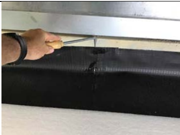
Probe testing the perimeter termination detailing.
