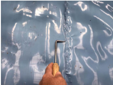
Probe testing all hand welded membrane laps.
