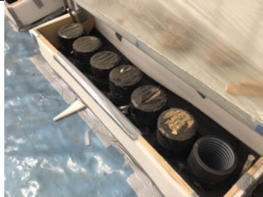
Pipe penetration detailing inside of a boxed off area.
