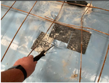
Recorded defects were patched repaired by installer using Juta GP1 SAM and probe tested.
