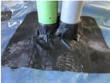
Pipe penetration detailing in unit 3 communal area.
