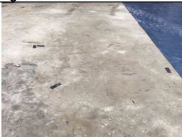
Evidence of the well rolled fine aggregate prior to the membrane being laid.
