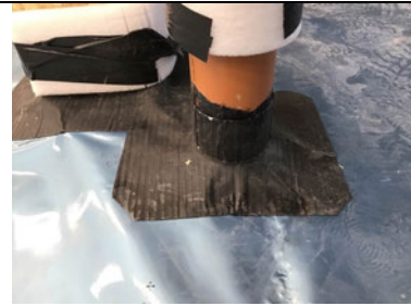
Typical pipe penetration detailing in the communal area in unit 2.
