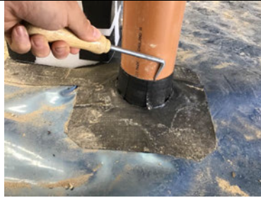
Probe testing a typical pipe penetration detail.
