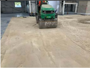
Substrate base being continuously rolled prior to gas barrier installation.
