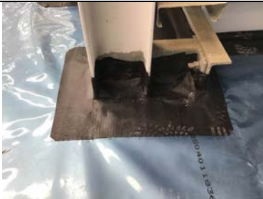
Typical steel stanchion detailing in unit 1.
