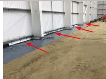
Miothene covering the perimeter detailing.
