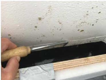
Probe testing a steel stanchion detail.
