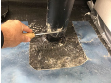
Probe testing a pipe penetration detail.
