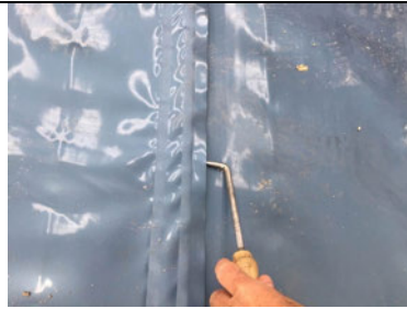
Probe testing an auto welded membrane lap.
