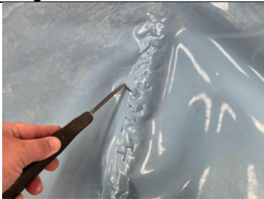
Probe testing along hand welded membrane lap joints.
