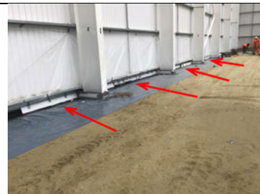
Miothene covering the perimeter detailing.
