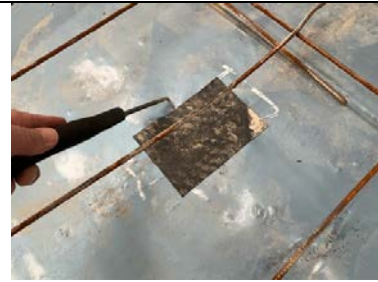
Recorded defects were patched repaired by installer using Juta GP1 SAM and probe tested.
