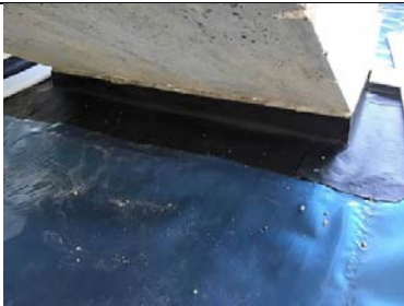
Base of concrete stair detailing.
