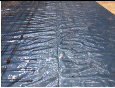
Overview of a hand welded membrane lap.
