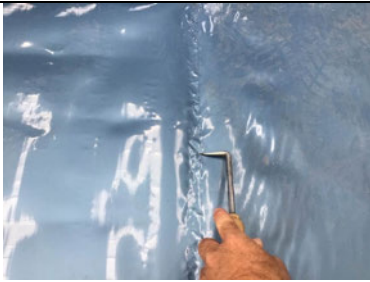
Probe testing a hand welded membrane lap.
