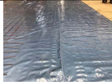
Overview of a auto welded membrane lap.
