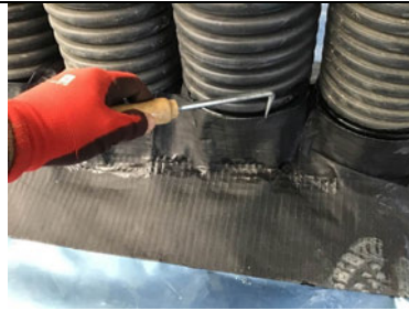
Probe testing all pipe penetration detailing in unit 2.
