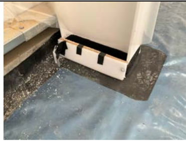
Restricted inspection to steel stanchions.
