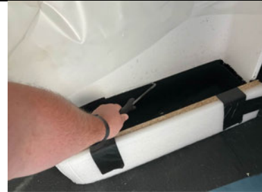
Probe testing to restricted steel stanchion.
