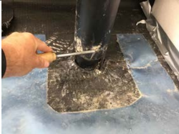
Probe testing a pipe penetration detail.
