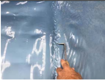
Probe testing a hand welded membrane lap.
