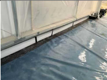
Overview of the restricted inspection to the retrofit
