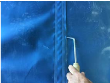
Probe testing the auto welded membrane lap.
