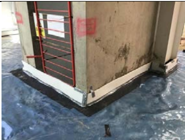
Miothene was placed around the lift pit at the time of our inspection.
