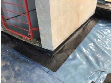
Retro fit detailing to the base of the concrete lift pit.
