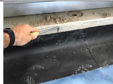
Probe testing the heat sealed perimeter curb stone detailing.
