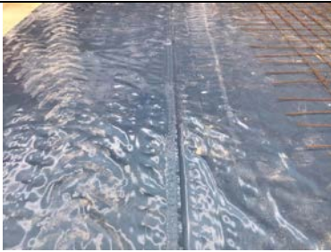
A typical auto welded membrane lap.
