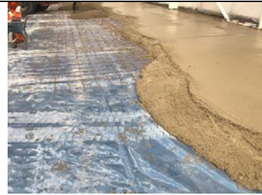
Overview of the Juta GP5 gas membrane being installed.
