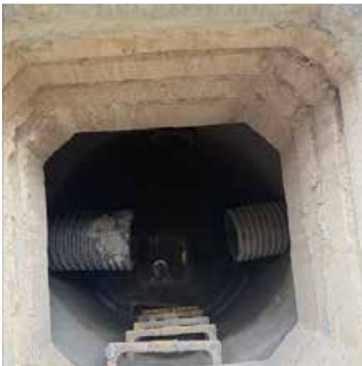
Existing surface water chamber before attenuation tank – IC.4 – May 2026 (Left hand connection from Unit 12a. Right hand connection from Unit 12.)
