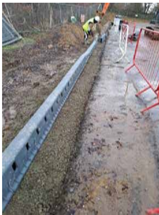
Car park / access road surface water drainage kerb - January 2024
