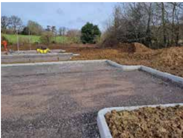
Car park permeable sub-base installed – February 2024
