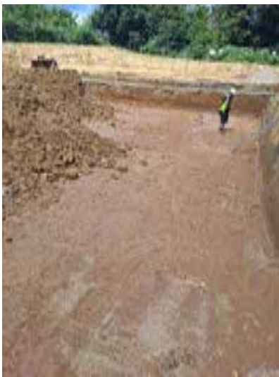
Attenuation tank excavation – August 2023
