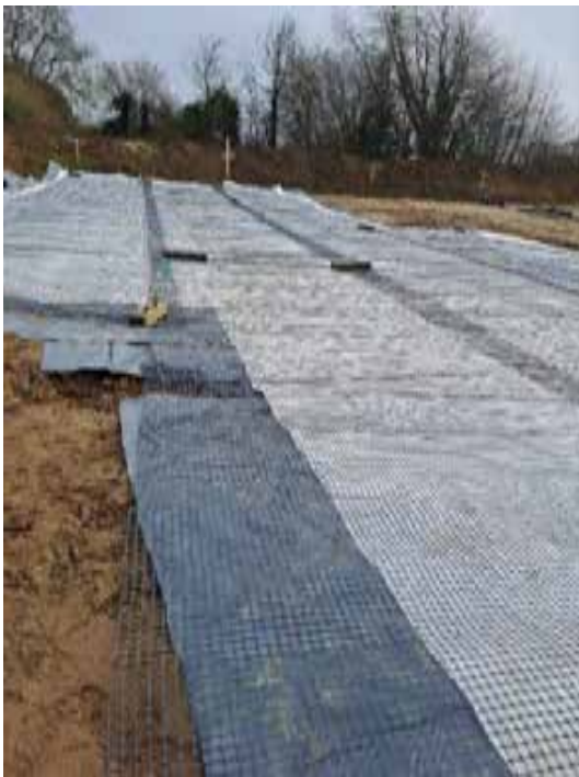
Carpark geotextile and sub-baffles in progress – January 2024
