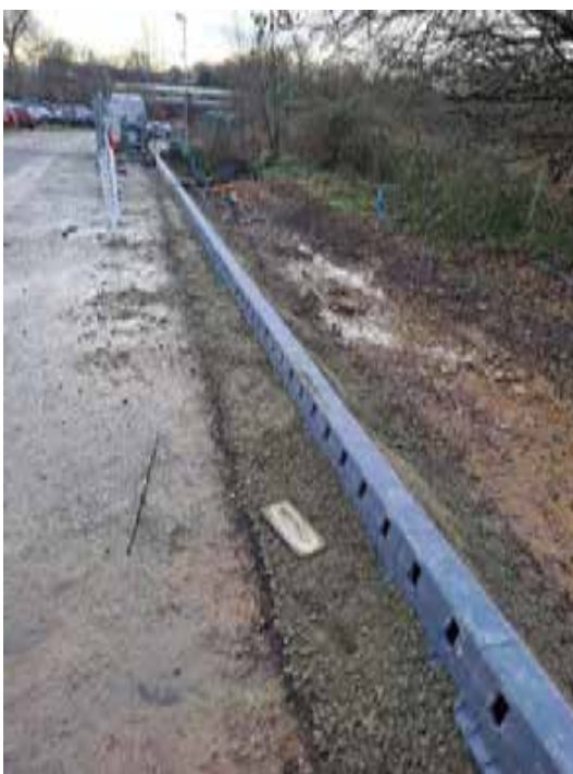
Car park / access road surface water drainage kerb - January 2024
