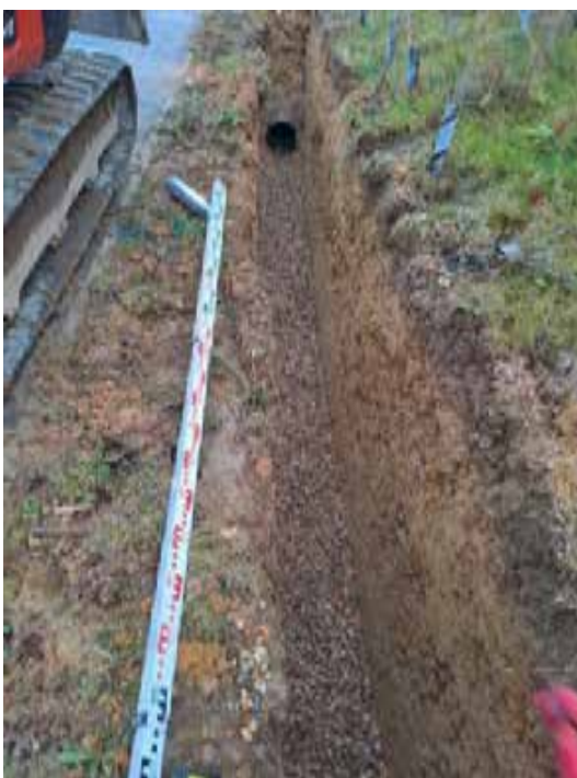
Connection to existing surface water - November 2023
