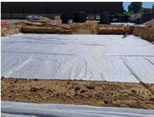
Attenuation tank, geotextile installation– September 2023
