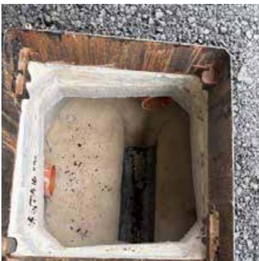
New surface water IC 6 & 7 – May 2026
