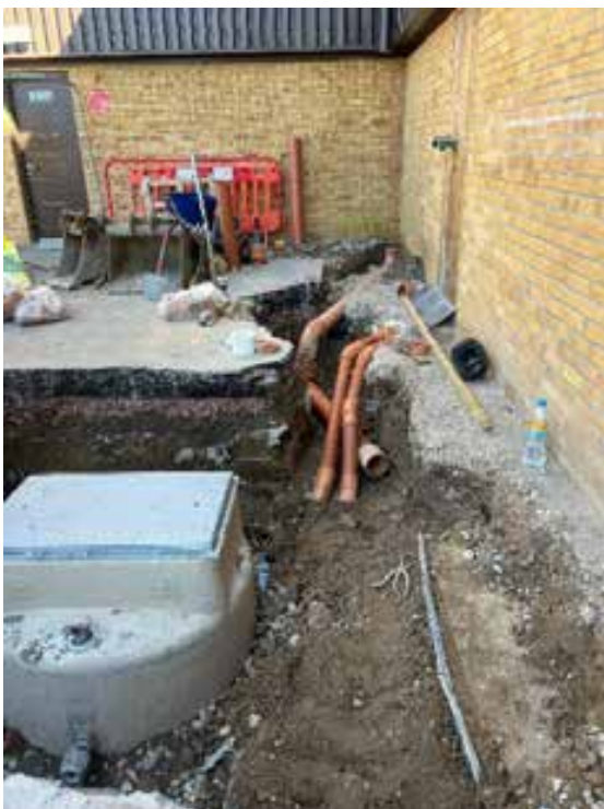
New Surface water drainage, below foul and past new pumped foul main – March 2026
