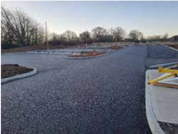
Carpark, permeable tarmac installed – March 2024
