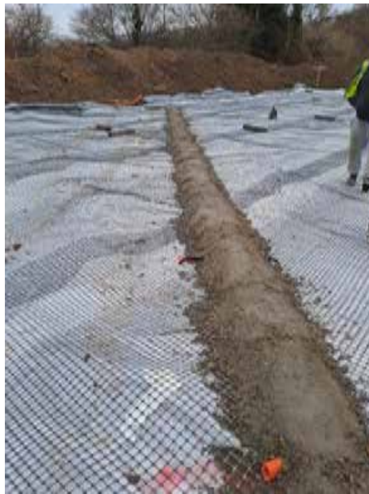
Carpark geotextile and sub-baffles in progress – January 2024
