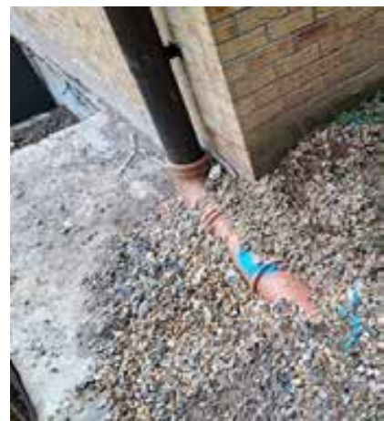
Rainwater connection of Unit 12 – temporary and permanent diversions of existing rainwater
