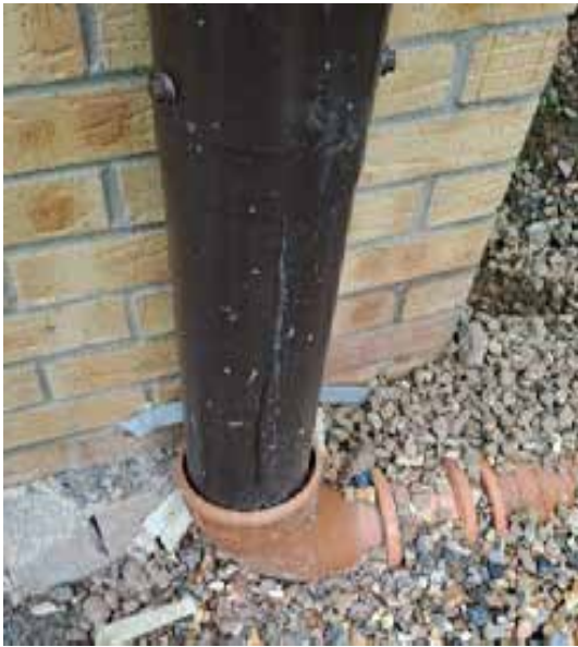
New surface water downpipe – May 2026
