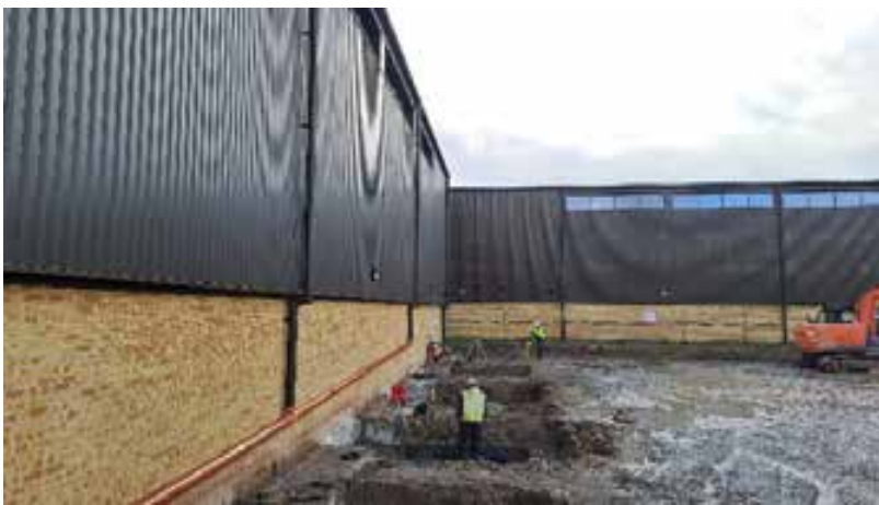
Rainwater connection of Unit 12 – temporary and permanent diversions of existing rainwater
