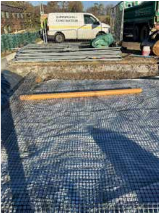
Geotextile membrane to car parking bays and permeable road at the rear /east Unit 12 – April 2026
