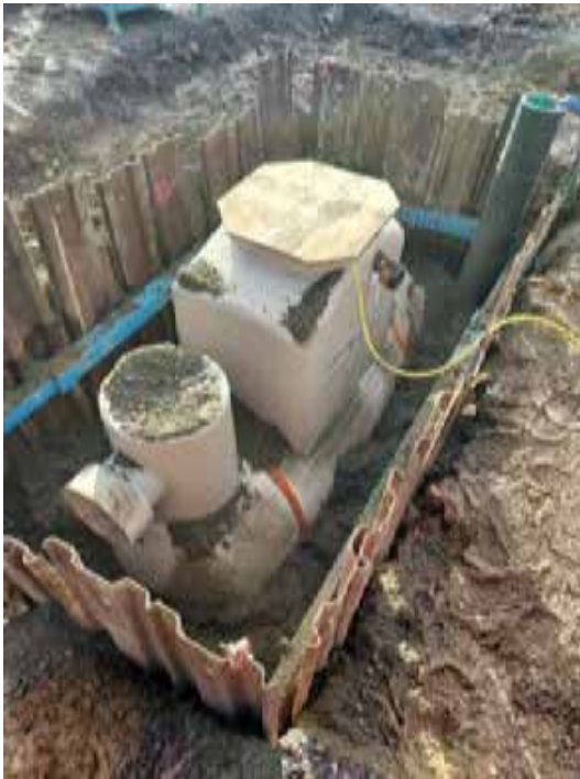
Klargester petrol interceptor tank installation - October 2023
