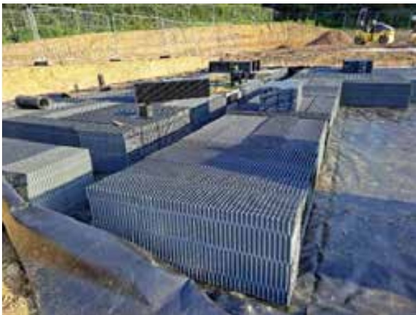
Attenuation tank, crate installation– September 2023
