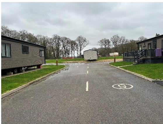
Entrance into the site from the south
