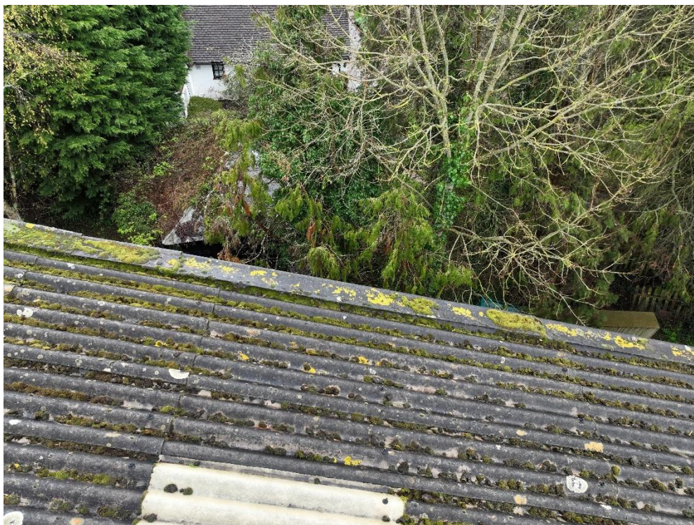
Photograph showing Prime Buildings roof and Great Daux Farmhouse in the background.
